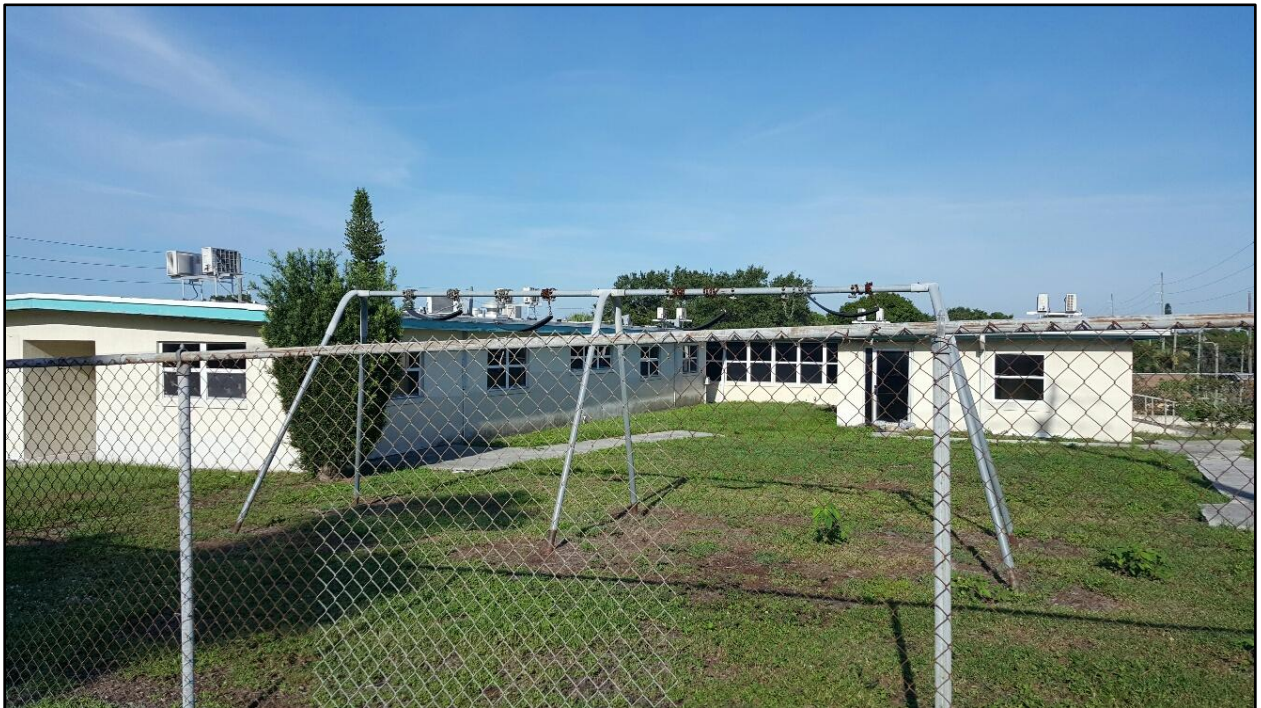
EXTERIOR VIEW OF SUBJECT IMPROVEMENTS
