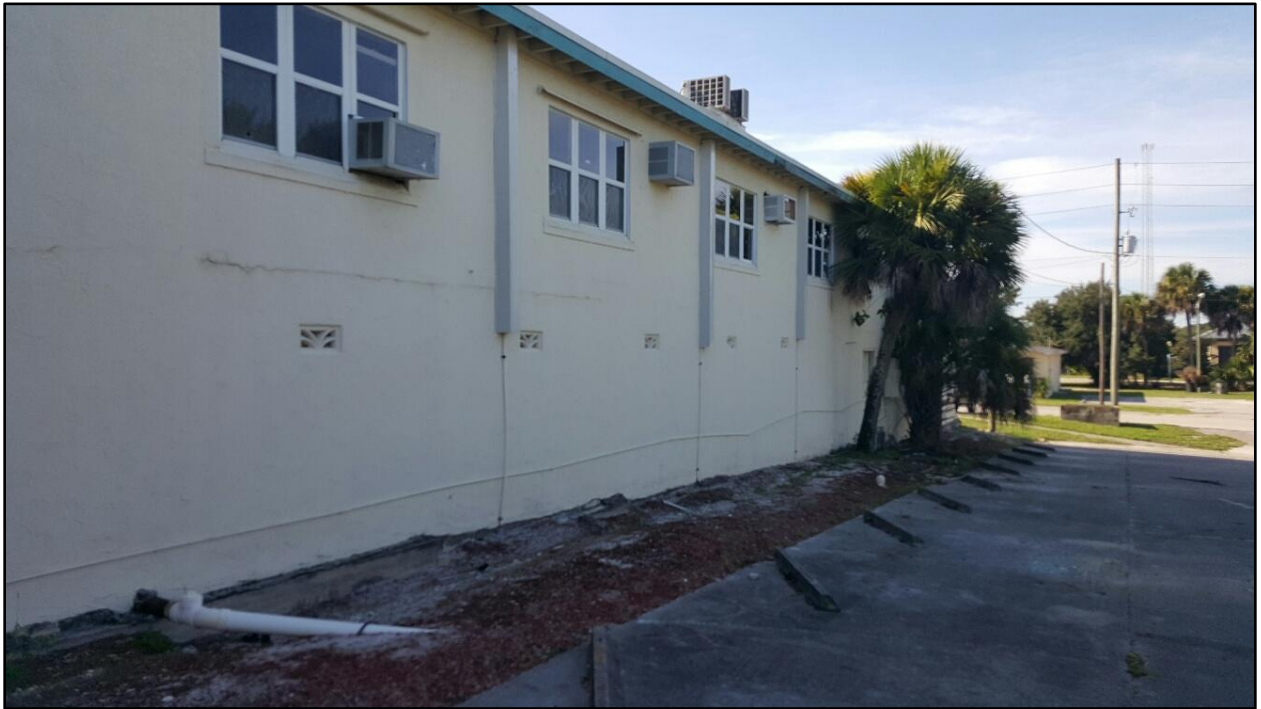
EXTERIOR VIEW OF REAR PORTION OF FACILITY
