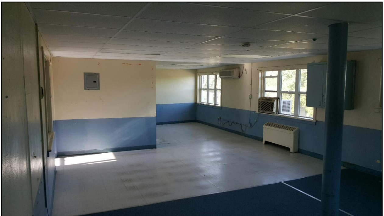
INTERIOR VIEW OF TYPICAL CLASSROOM AREA
