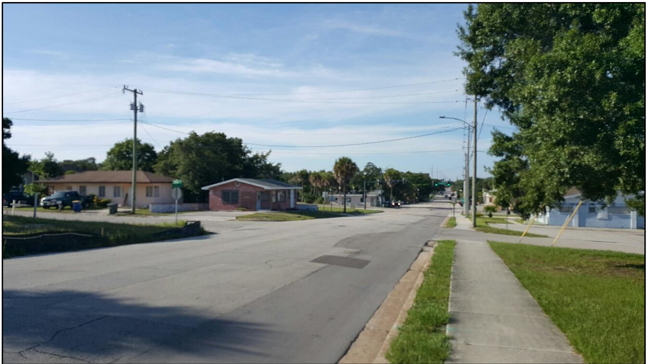
VIEW OF NORTH 7 TH STREET ON EAST SIDE OF SUBJECT
