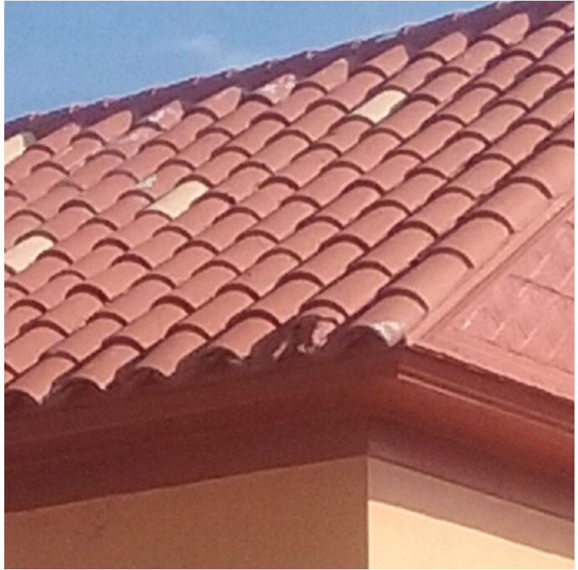
View of the existing barrel tile
