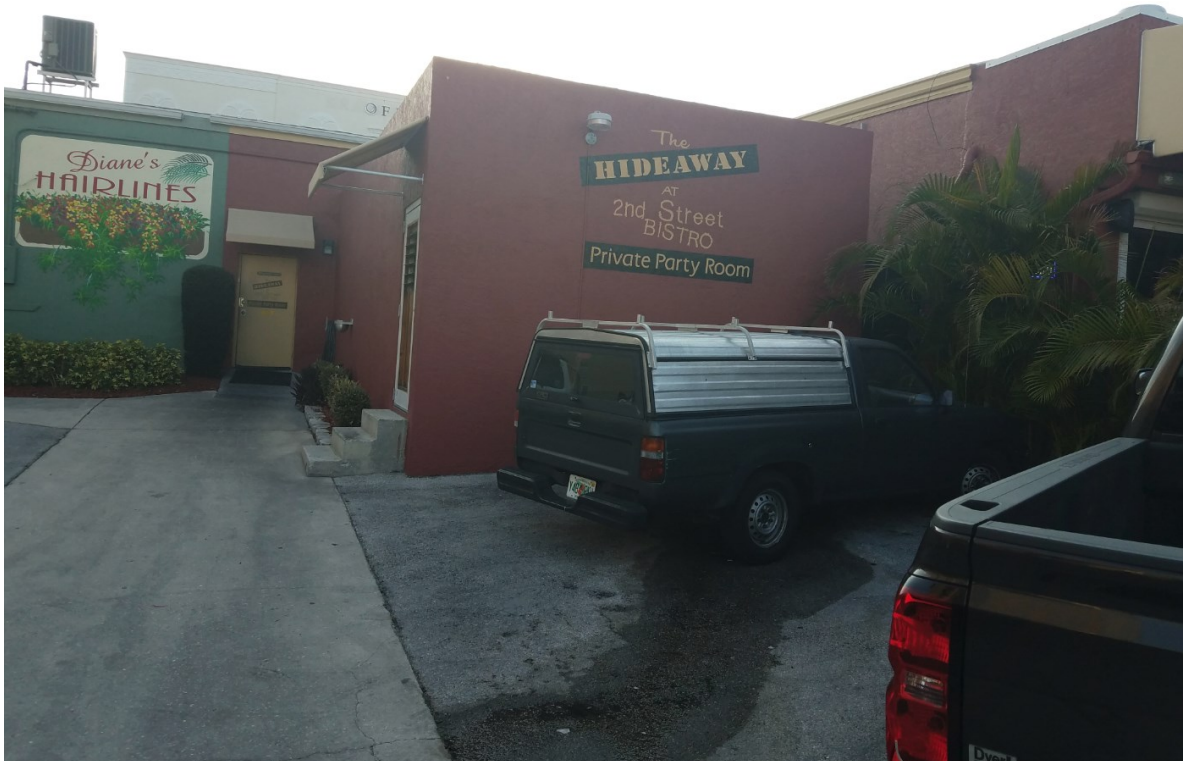
Existing site conditions
