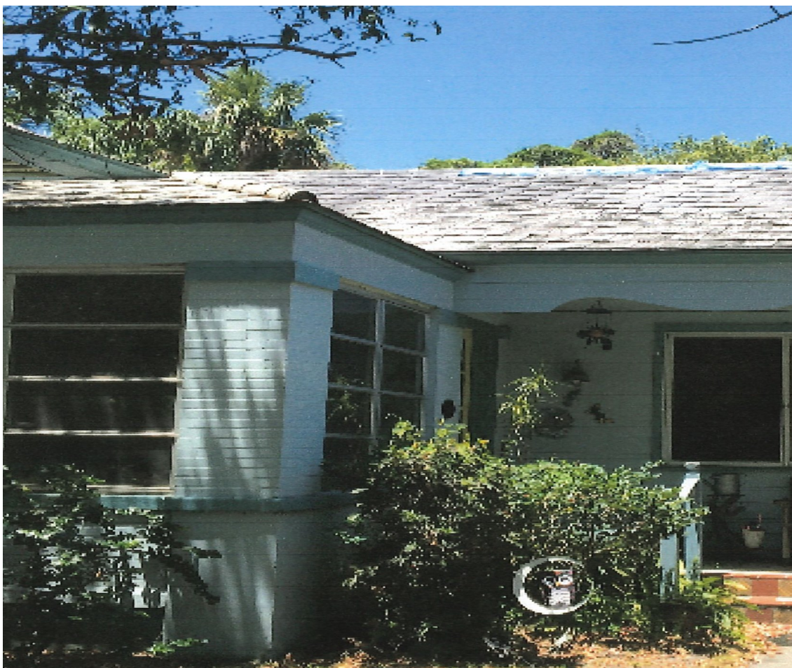
View of the existing asbestos shingle roof
