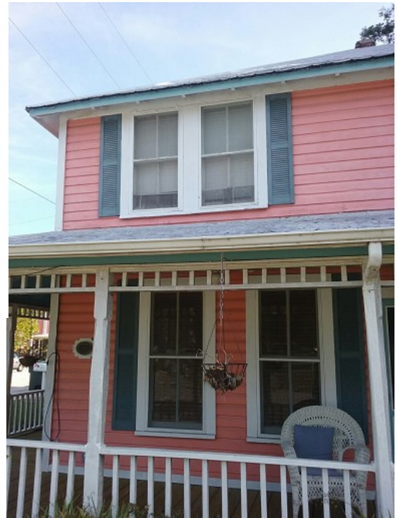
View of the existing windows
