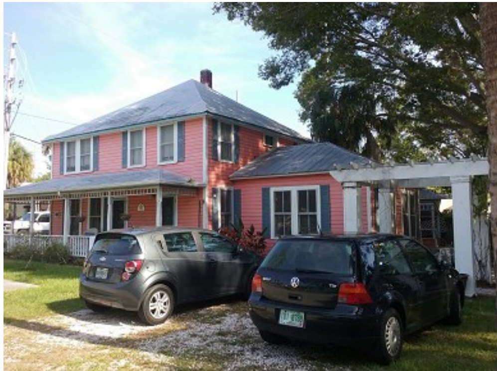
Cedar Place Facade
