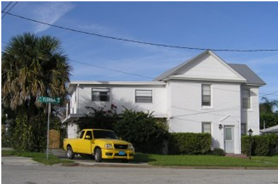
South/Florida Avenue Façade
