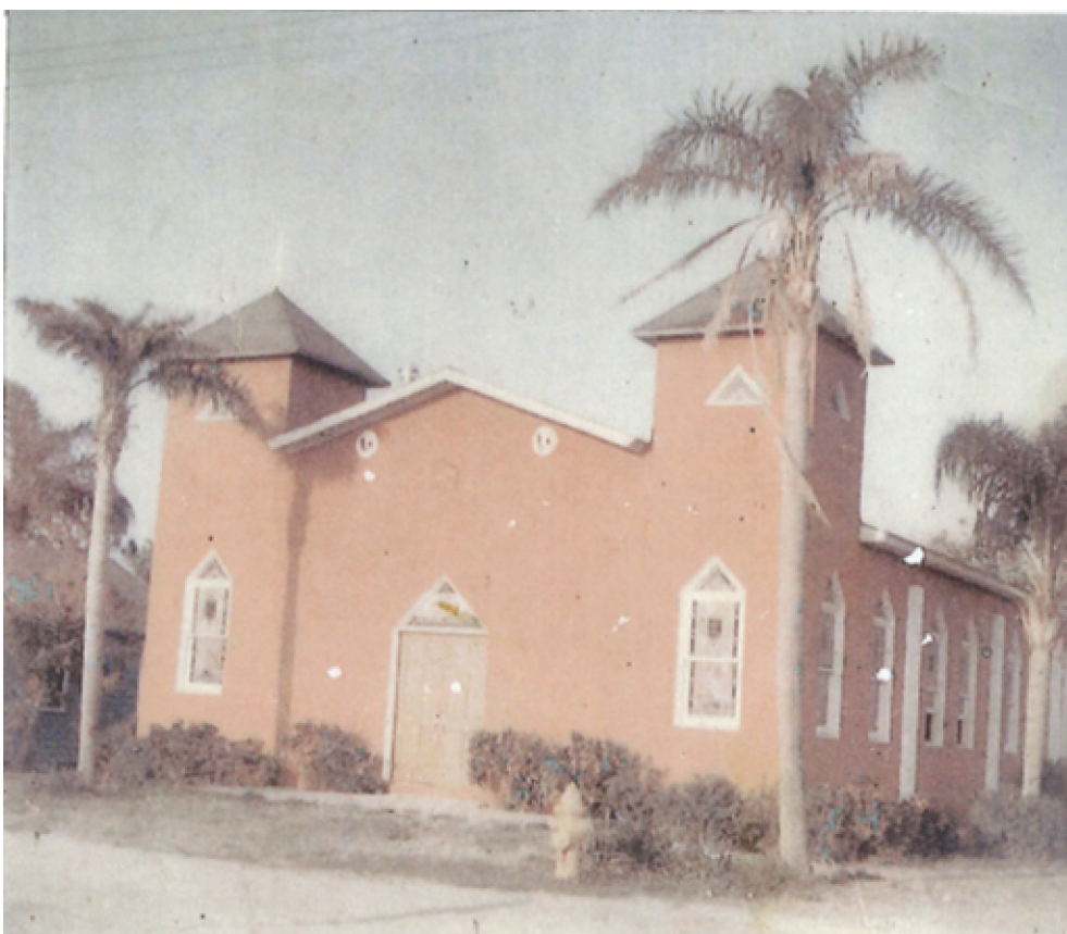
Original Front Façade
