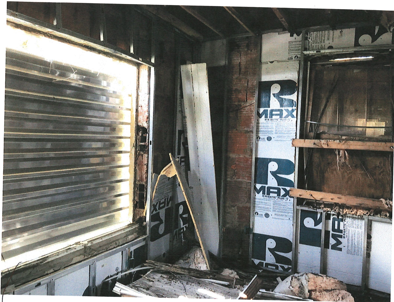
→ Front window, upstairs bedroom
