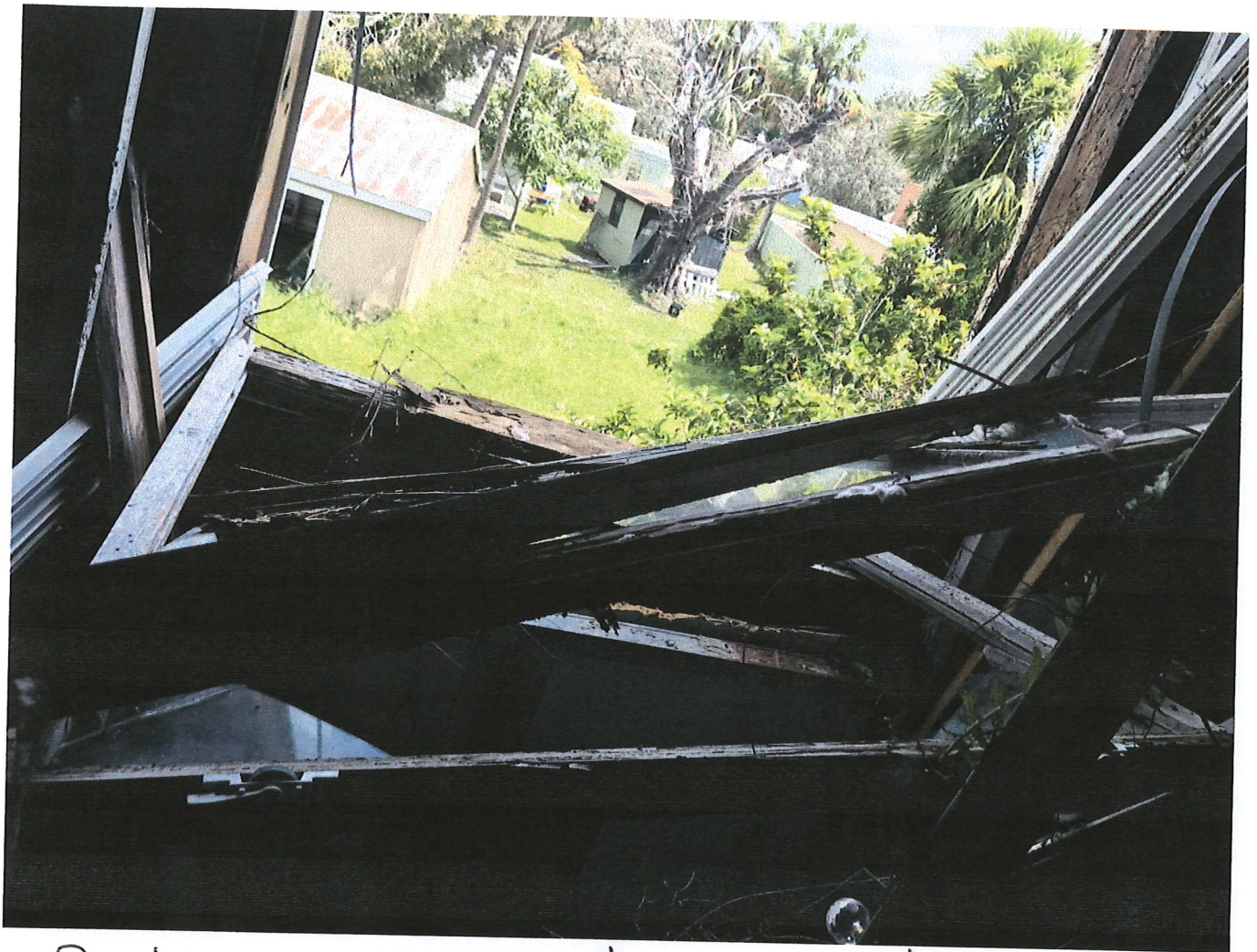
Back elevation bedroom window
