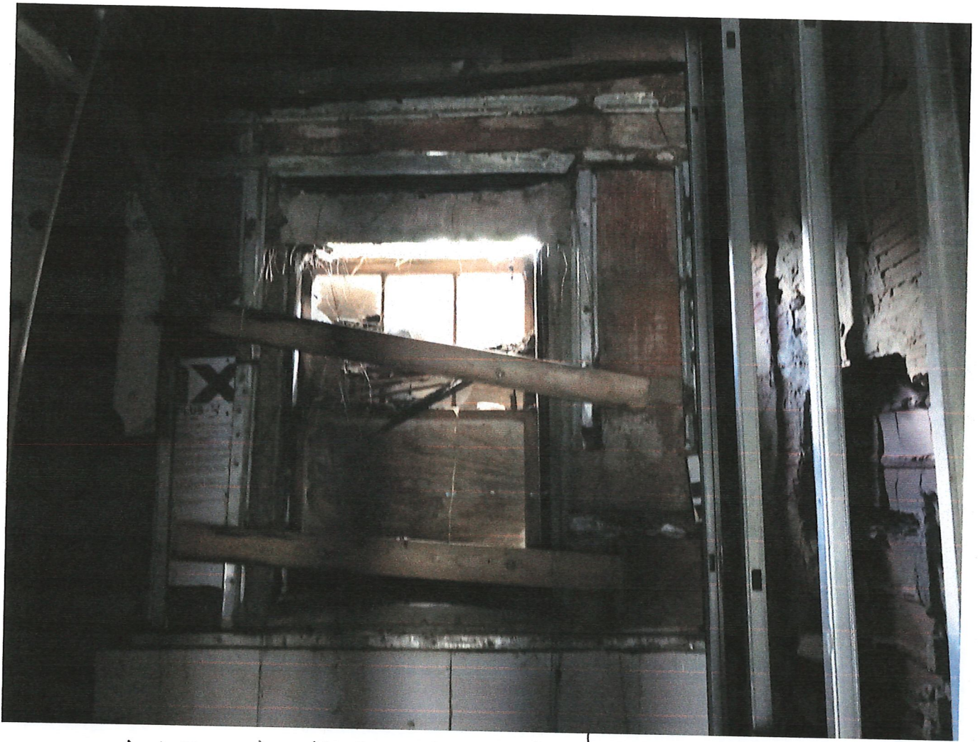
upstairs bathroom, window
