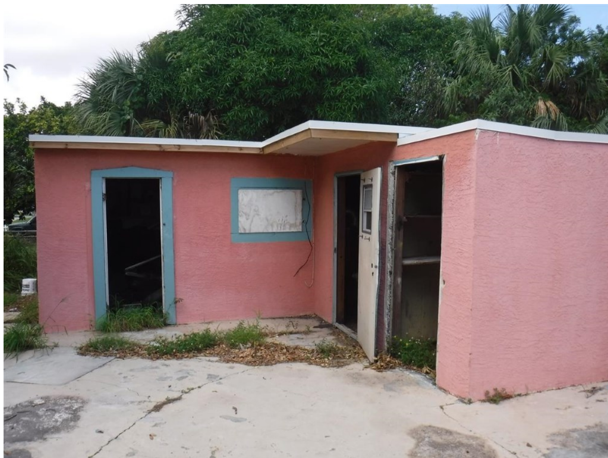
View of the subject structure
