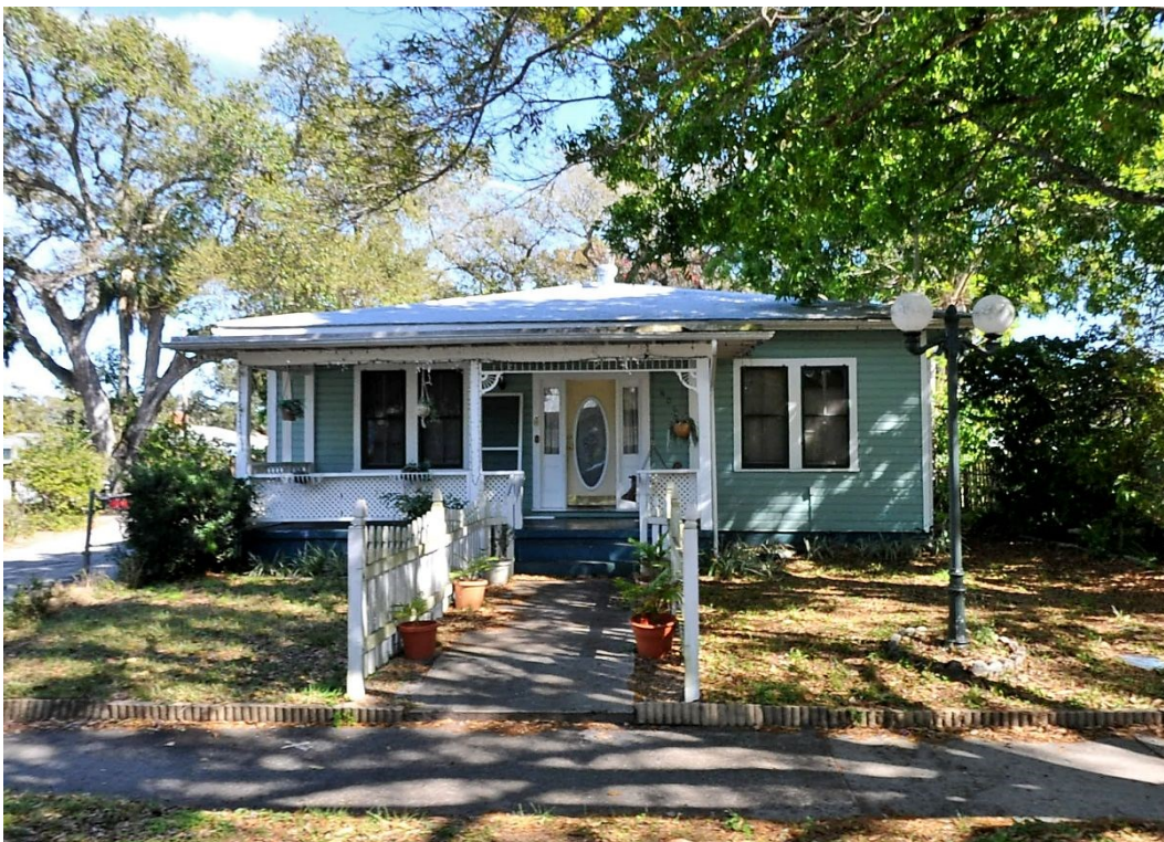
8th Street façade
