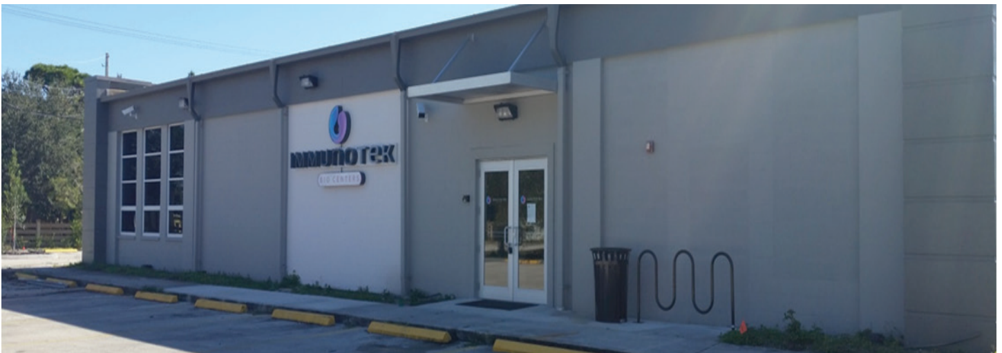
2710 S US Hwy 1- The Immunotek plasma donation center is nearing completion. Signage and landscaping has recently been installed. Final inspections should be scheduled in the near future. This picture was taken during a tie beam inspection.
