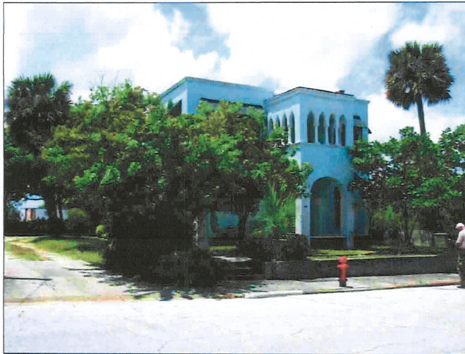
Contributing resource to the district: SL826, facing northwest (PCI May 2010).
