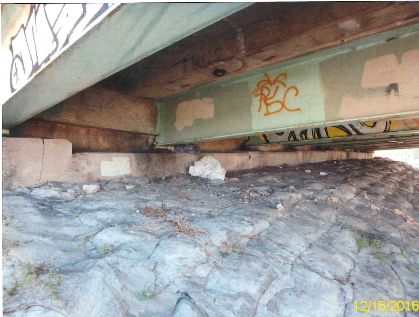
Photo 10 - Element 215 Re Conc Abutment
