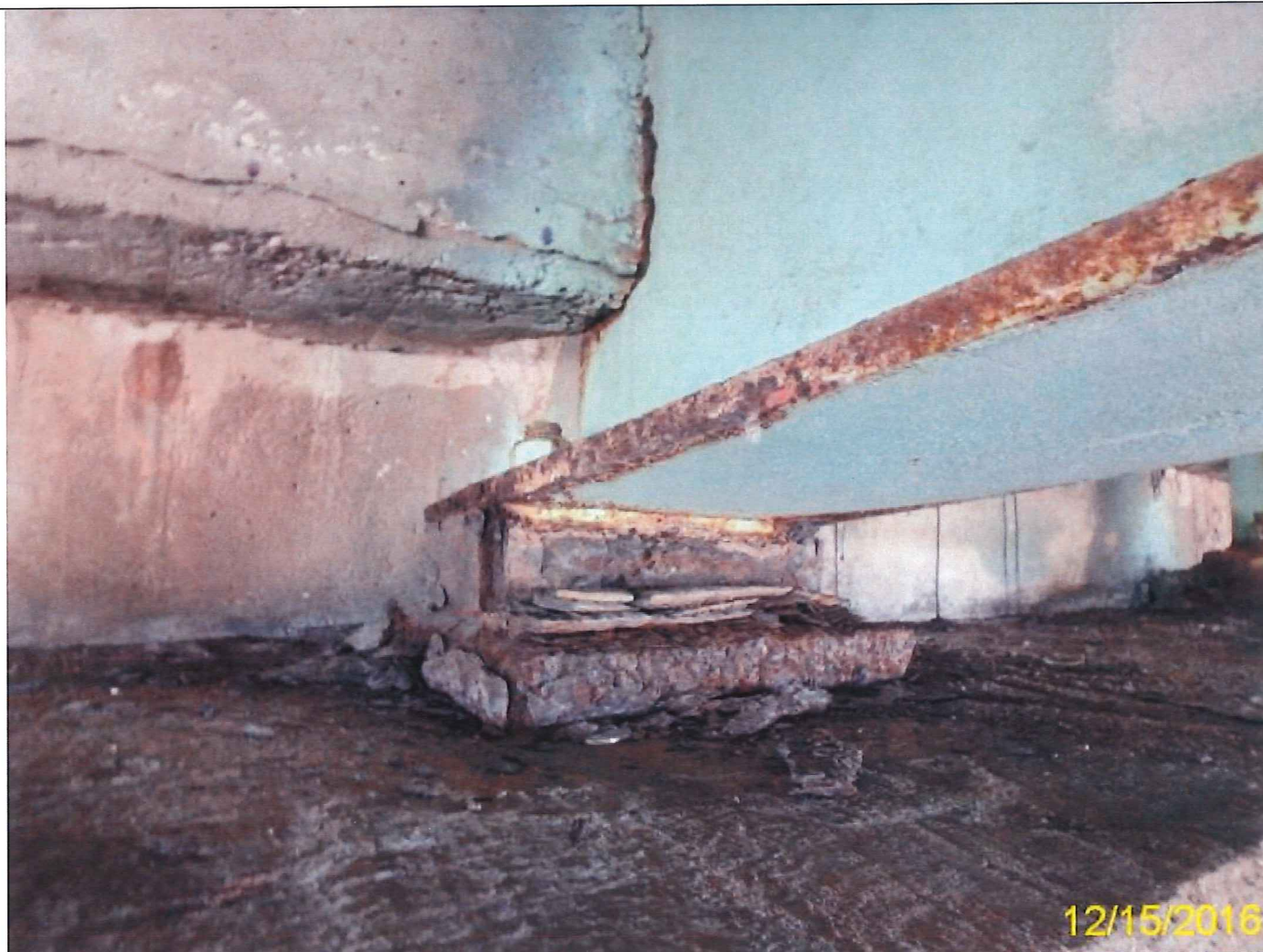
Photo 18 - Element 313 Fixed Bearing
