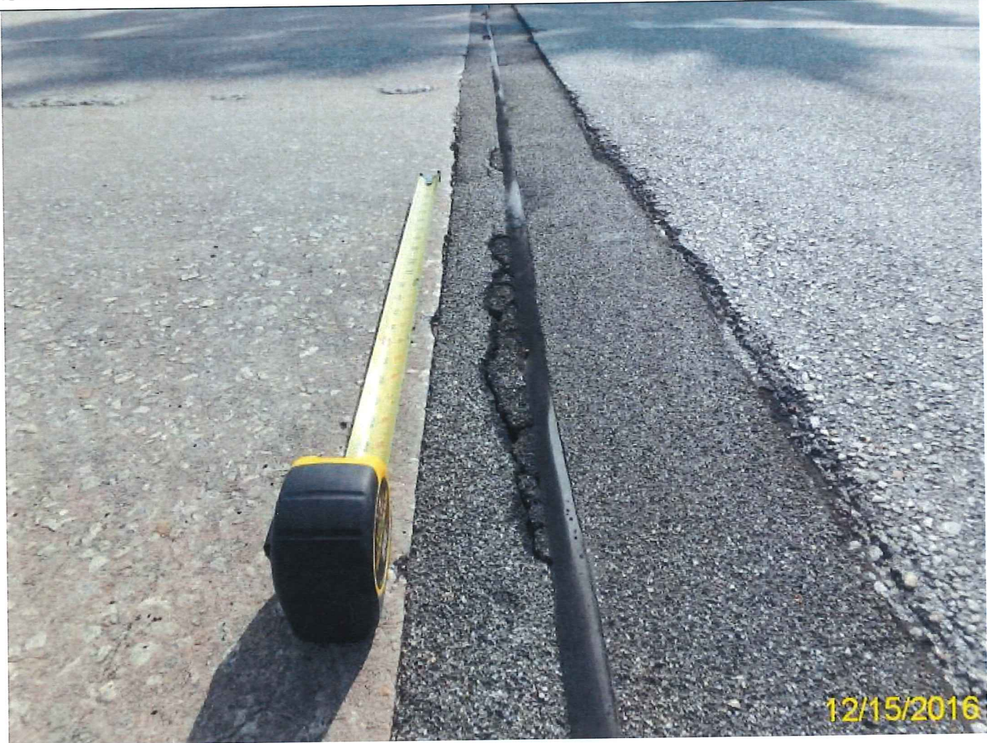
Photo 6 - Element 301 Pourable Joint Seal
