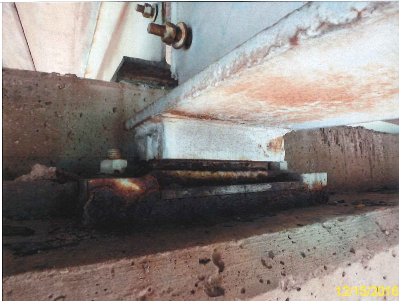
Photo 14 - Element 311 Moveable Bearing
