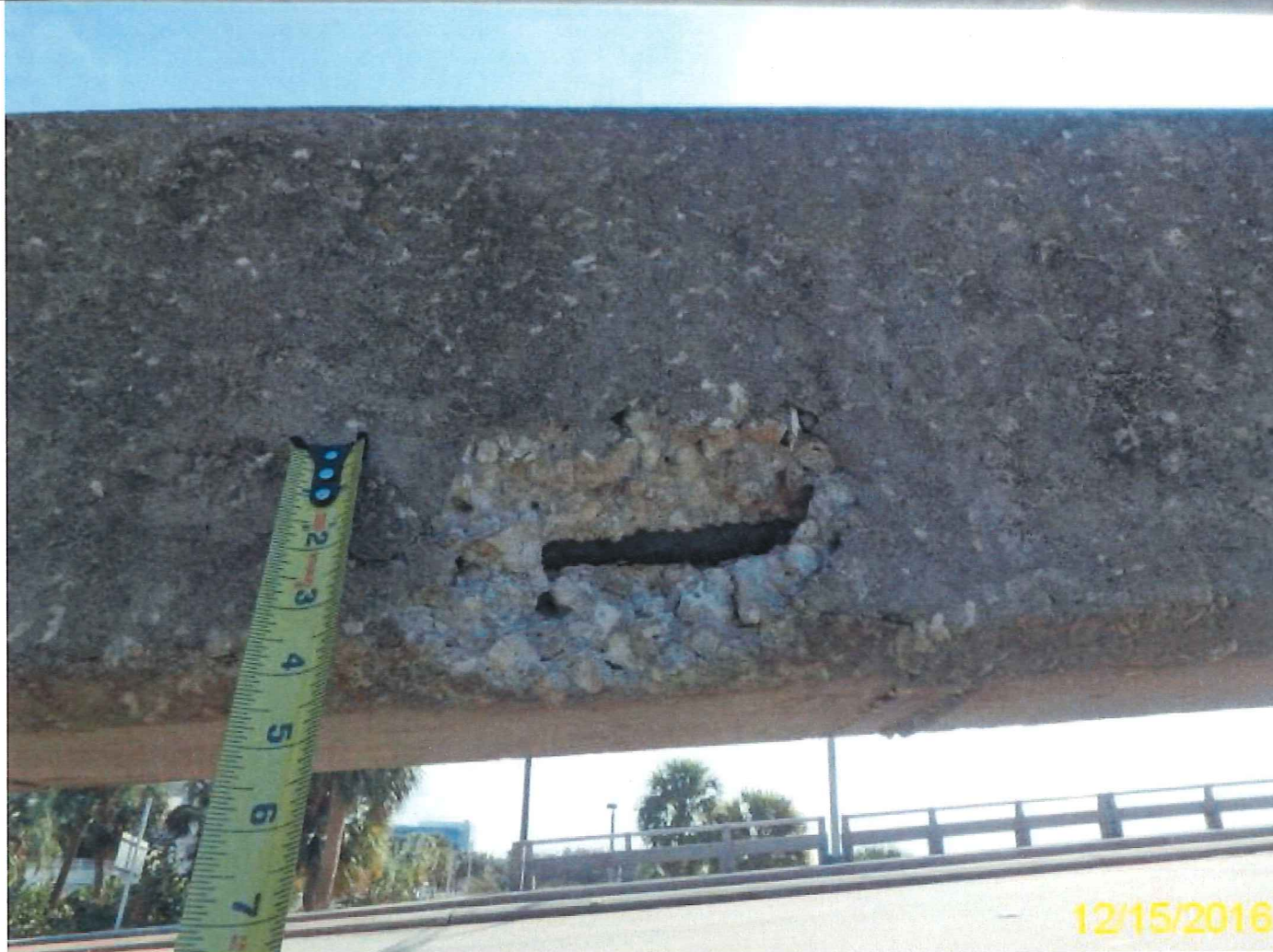
Photo 25 - Element 333 Other Bridge Railing
