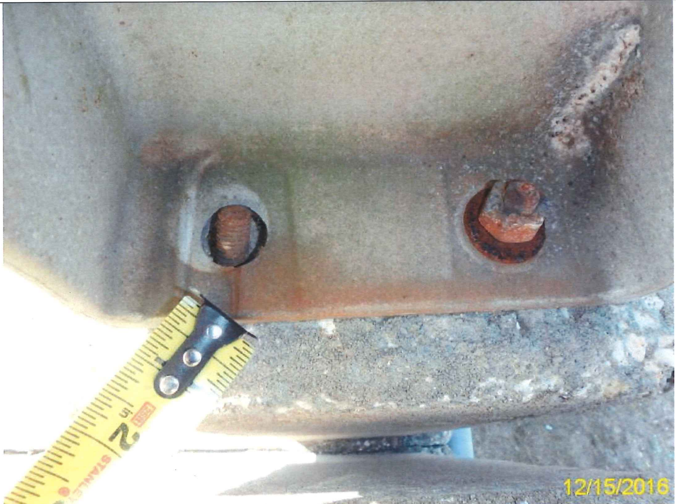
Photo 26 - Element 333 Other Bridge Railing
