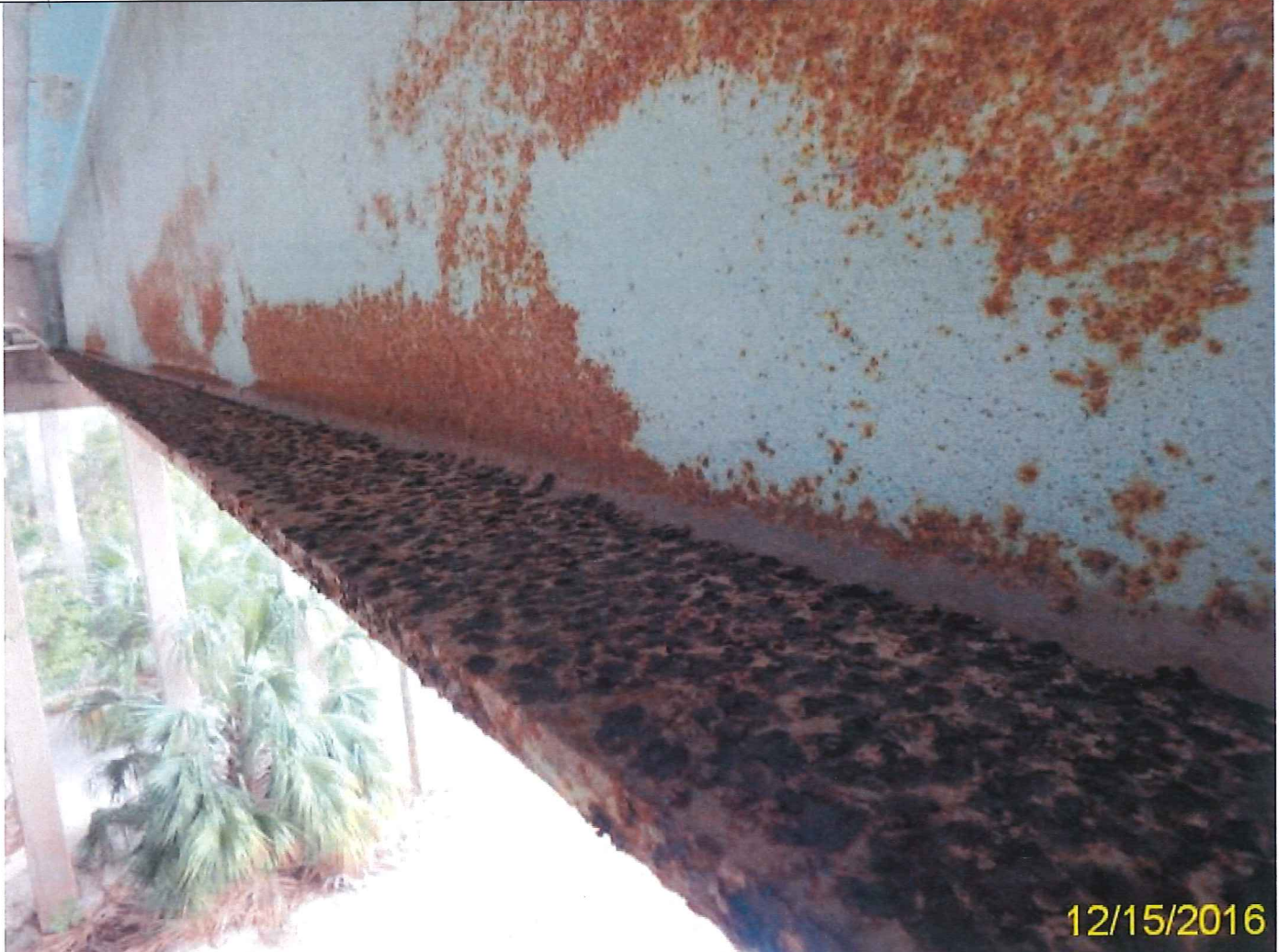
Photo 23 - Element 107 Steel Opn Girder/Beam
