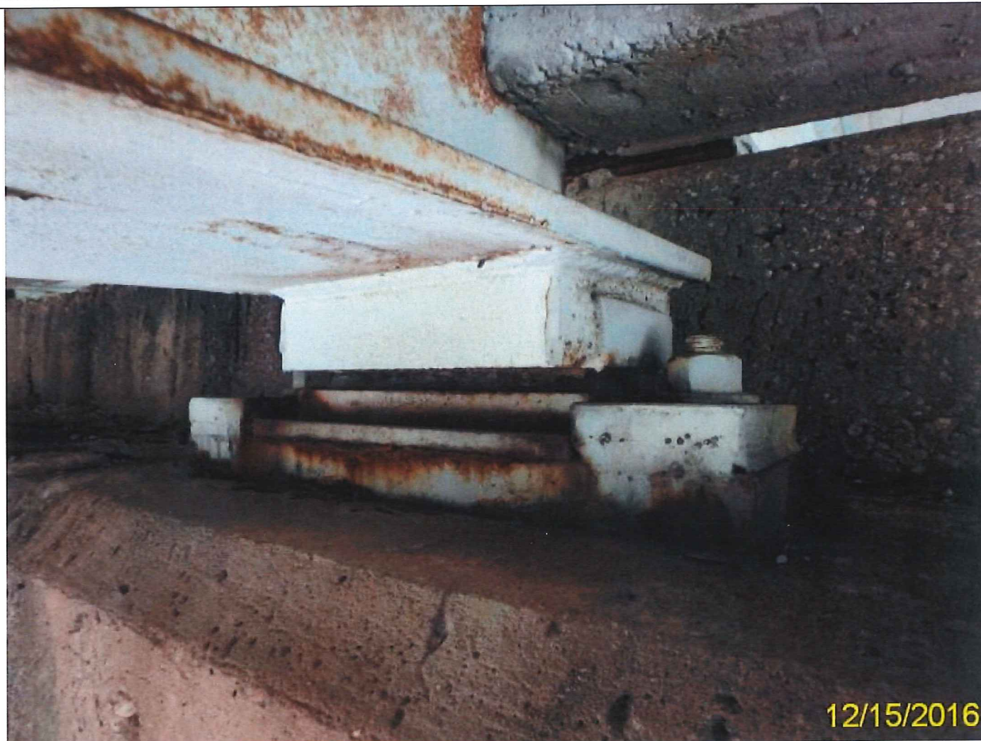
Photo 15 - Element 311 Moveable Bearing
