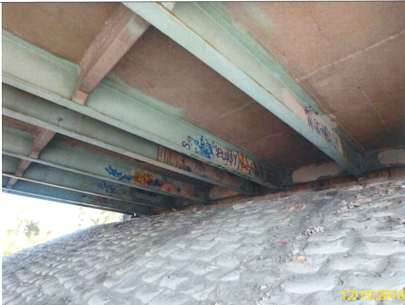
Photo 24 - Element 107 Steel Opn Girder/Beam
