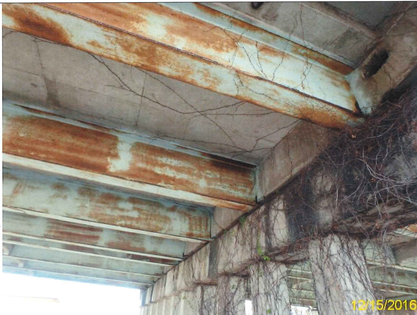
Photo 22 - Element 107 Steel Opn Girder/Beam
