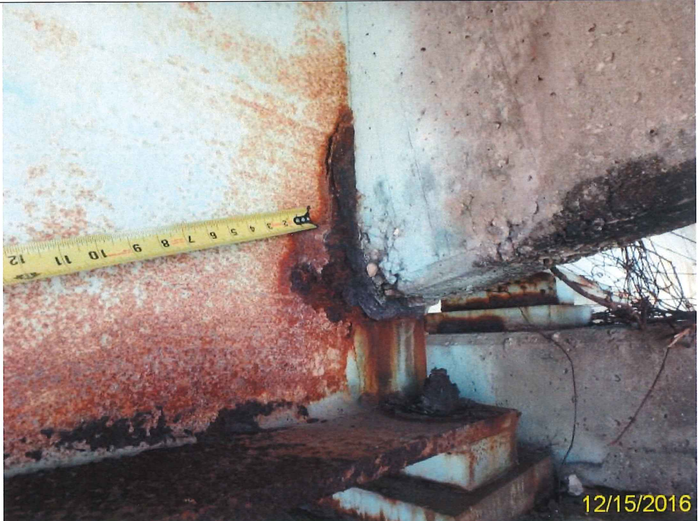
Photo 20 - Element 107 Steel Opn Girder/Beam
