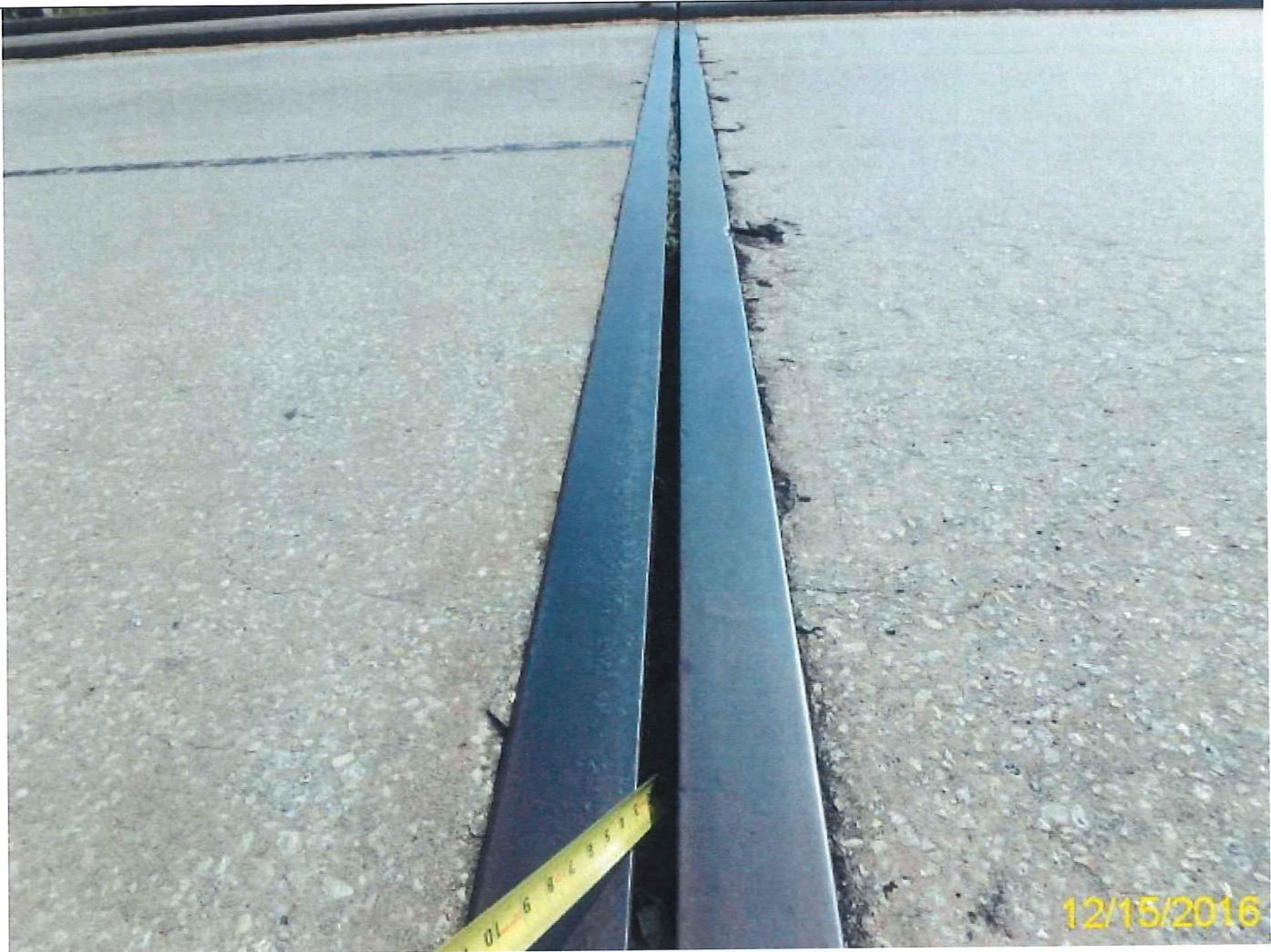
Photo 7 - Element 302 Compressn Joint Seal
