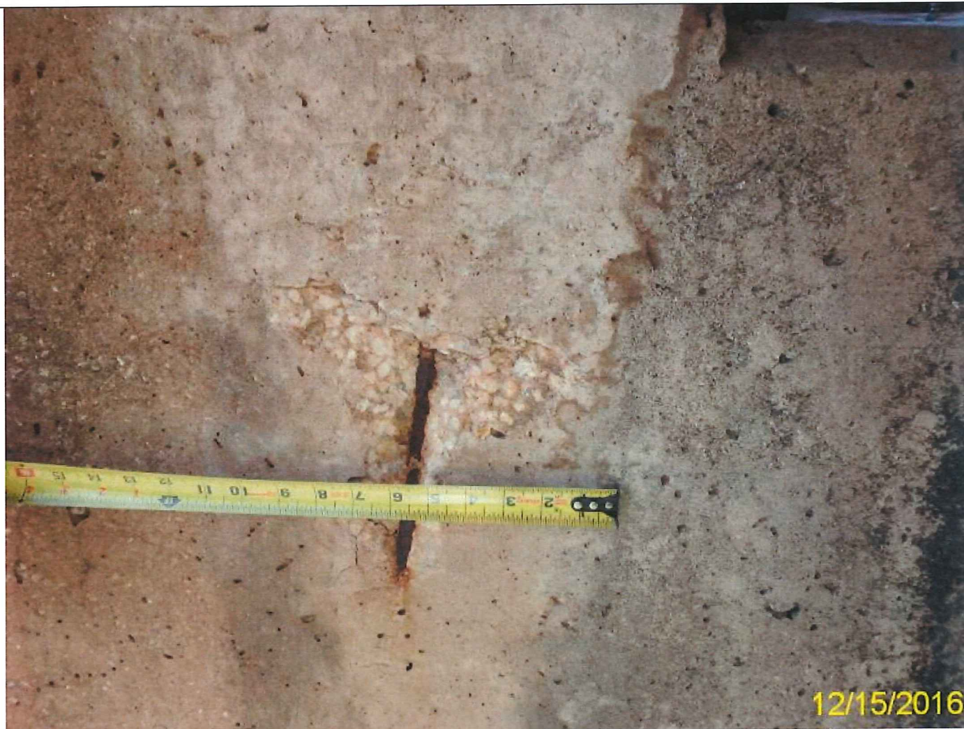
Photo 13 - Element 234 Re Conc Pier Cap
