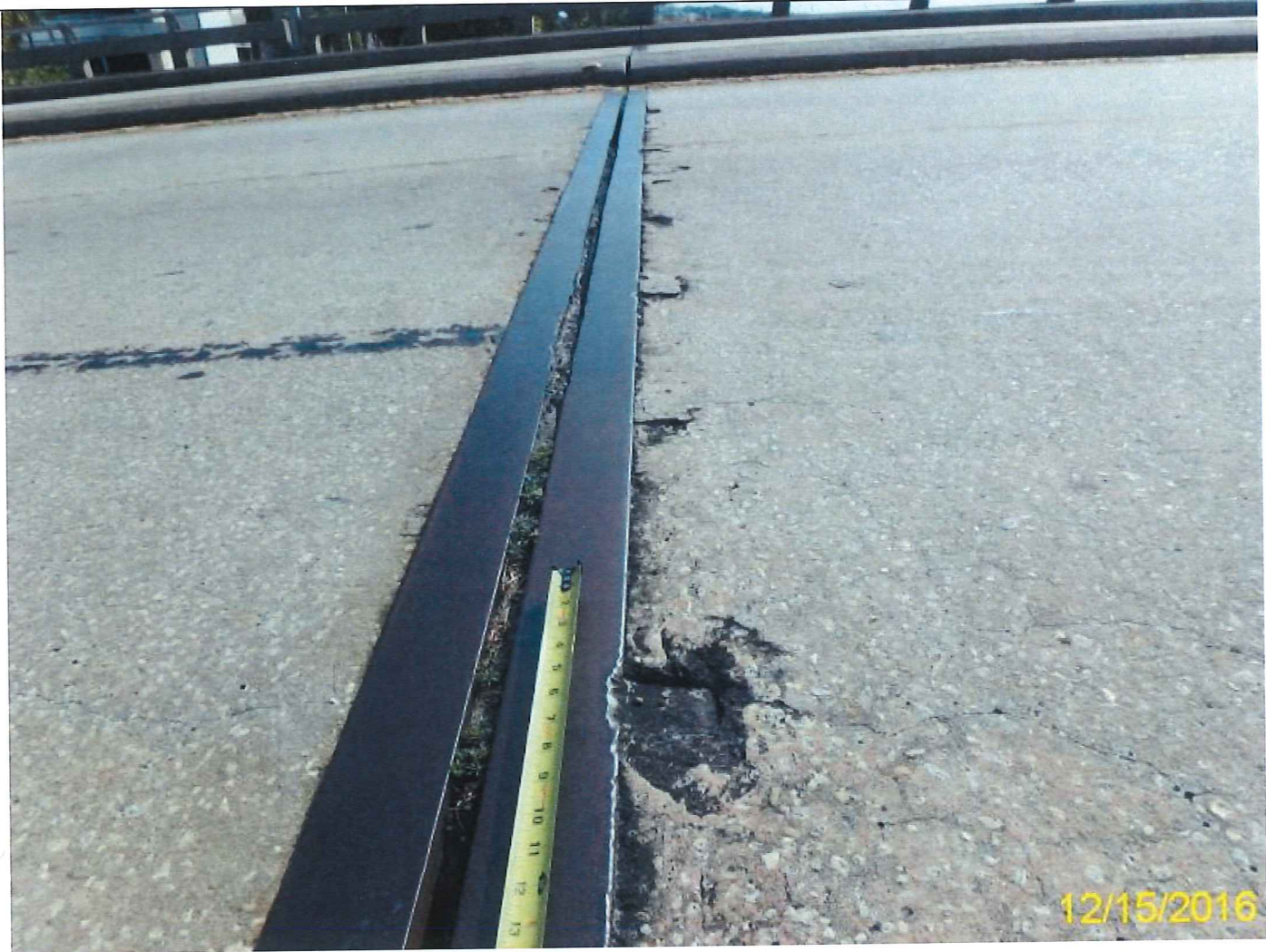
Photo 3 - Element 12 Re Concrete Deck
