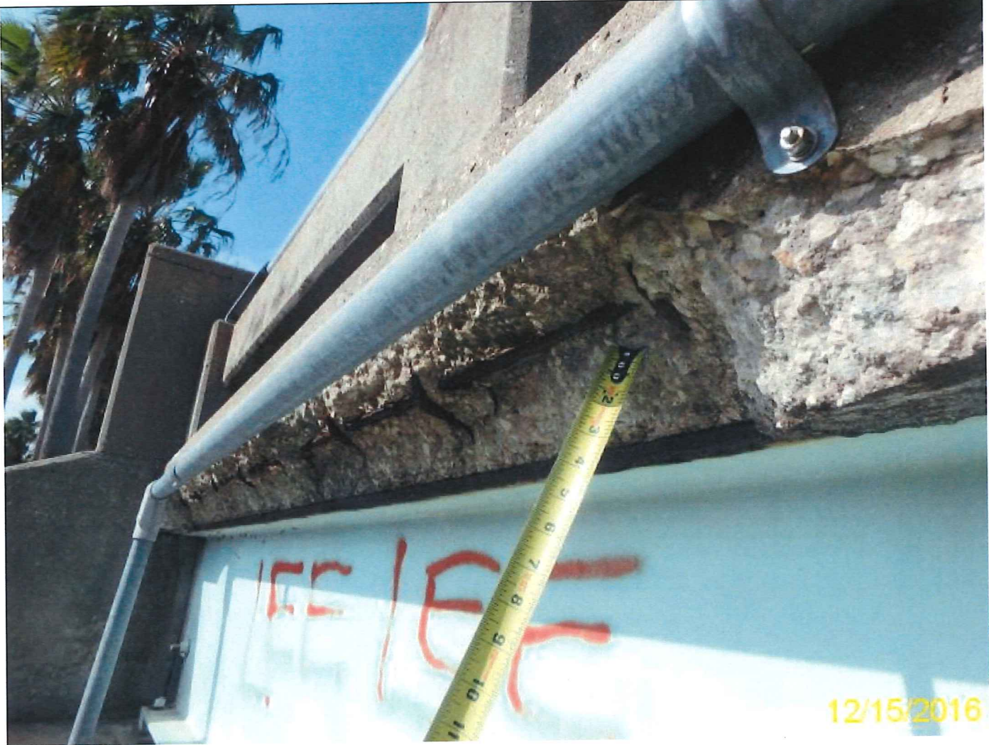
Photo 1 - Element 12 Re Concrete Deck
