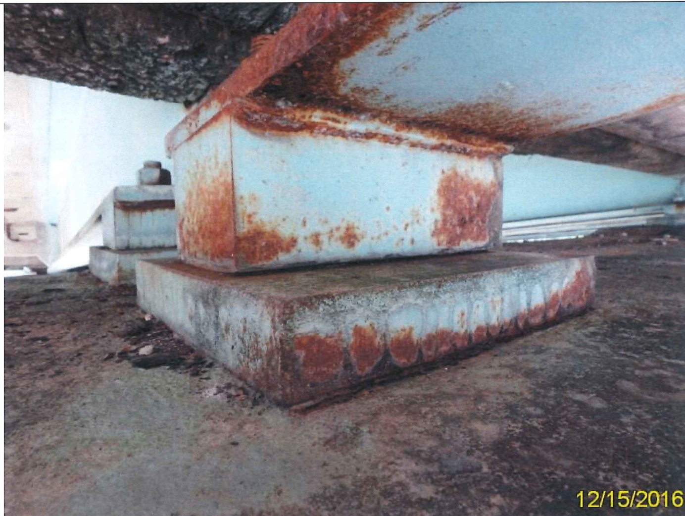
Photo 19 - Element 313 Fixed Bearing
