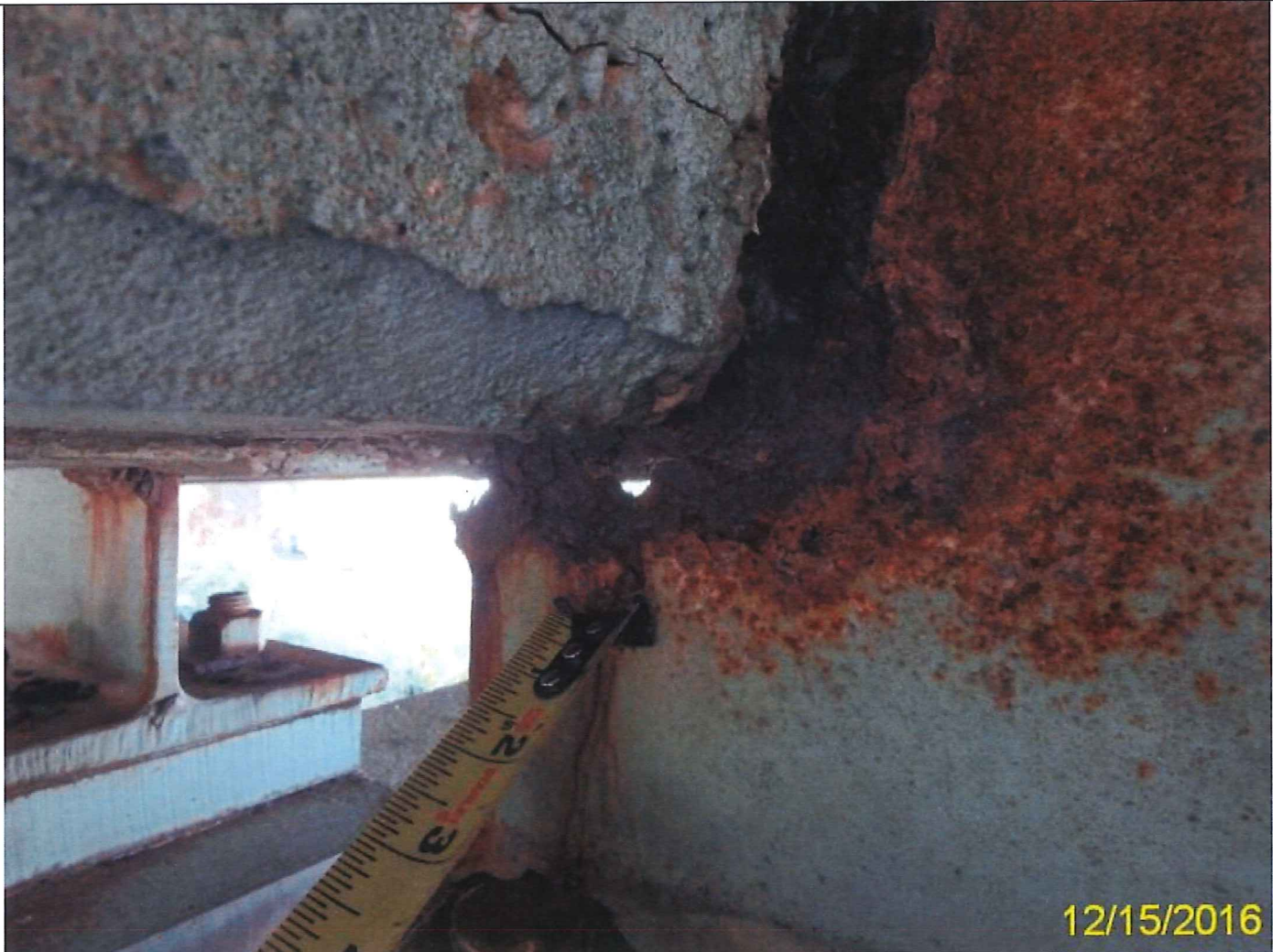
Photo 21 - Element 107 Steel Opn Girder/Beam
