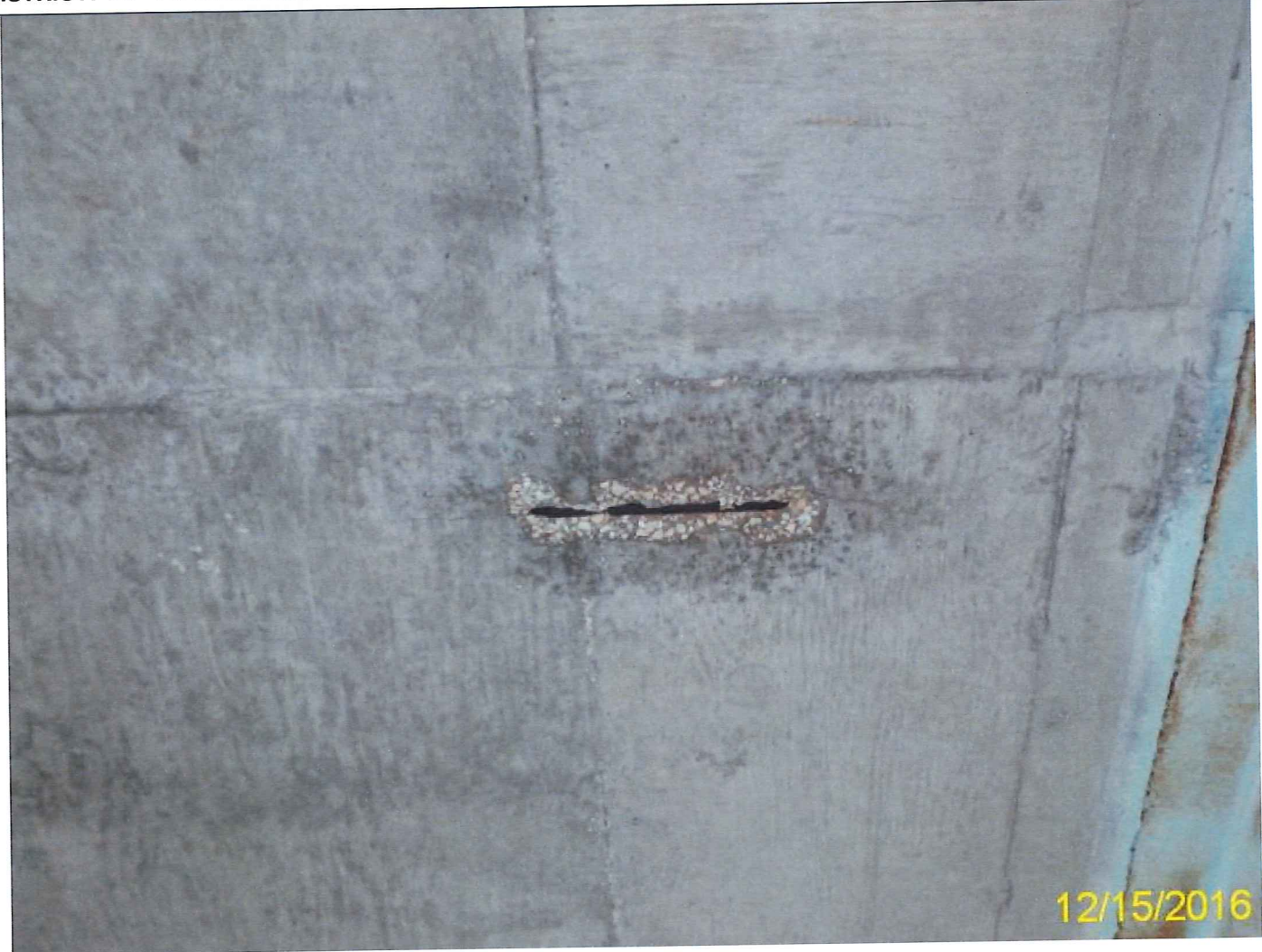
Photo 4 - Element 12 Re Concrete Deck
