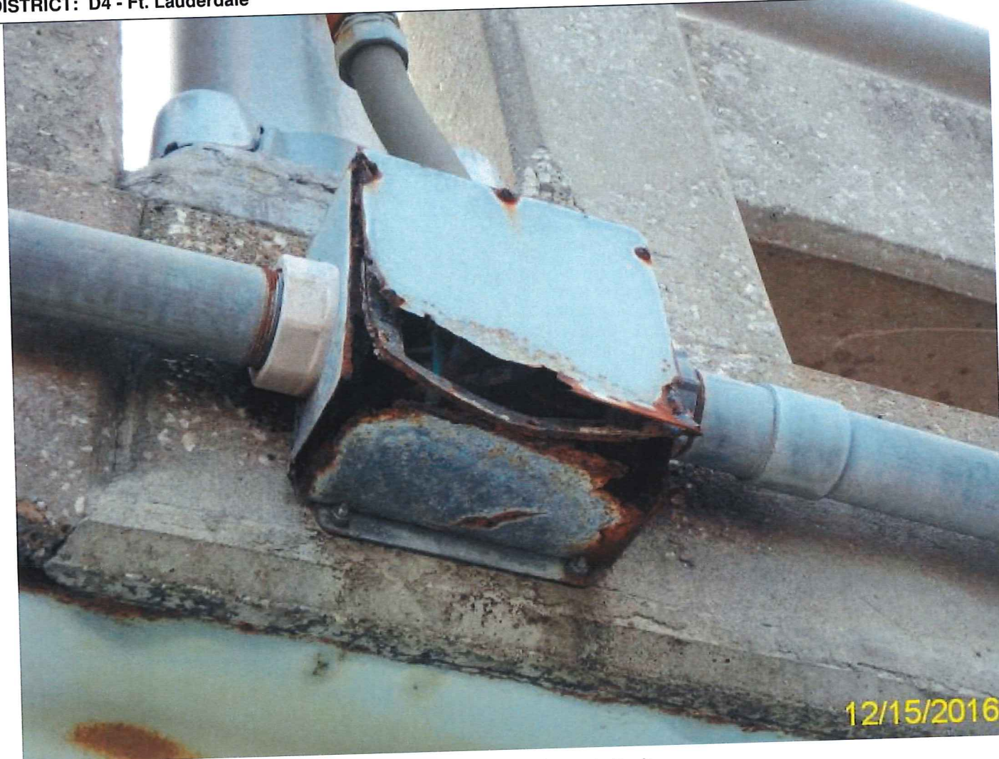
Photo 5 - Element 12 Re Concrete Deck
