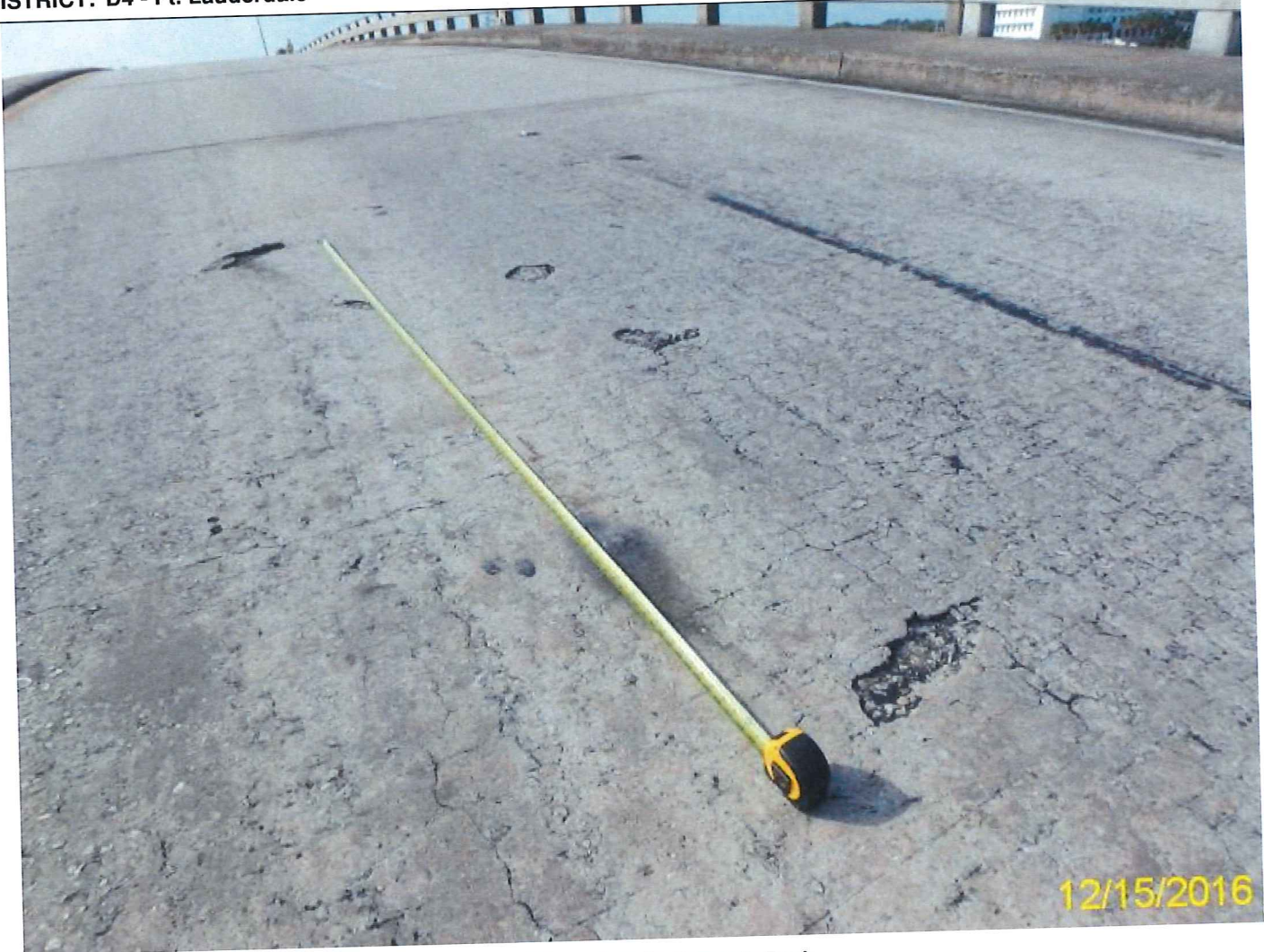
Photo 2 - Element 12 Re Concrete Deck
