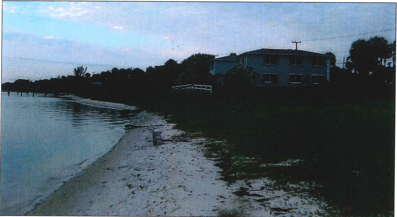
Photo looking south at strip of wetlands along shoreline of 401, 411, and 426 S. Indian River Drive.
