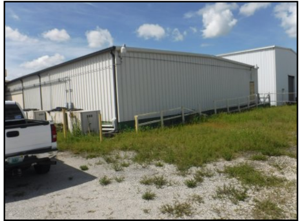
50 : Overview of citrus processing building, looking southwest
