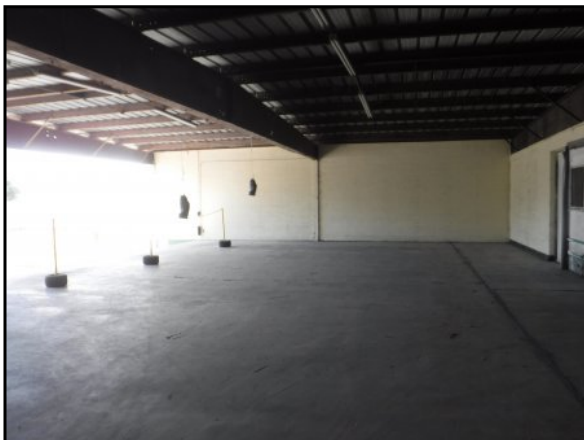
17 : Loading dock area in the citrus processing building
