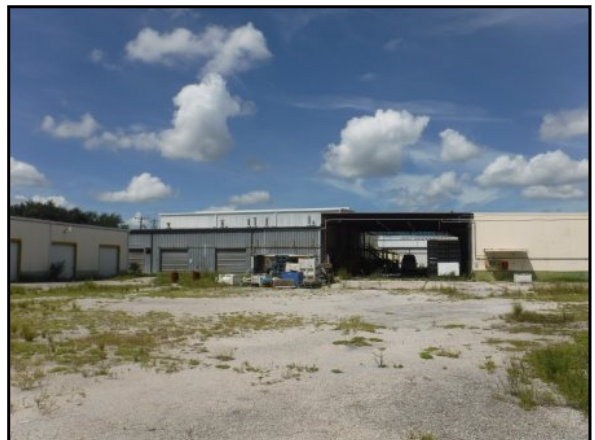
36 : Citrus processing building, looking southwest
