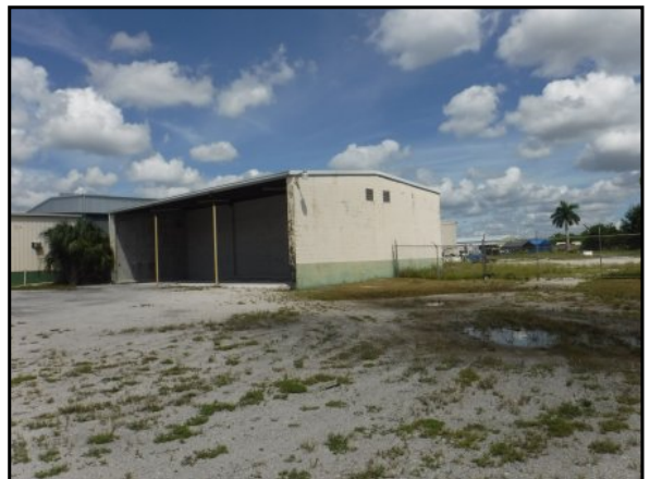
66 : Eastern elevation of the storage building
