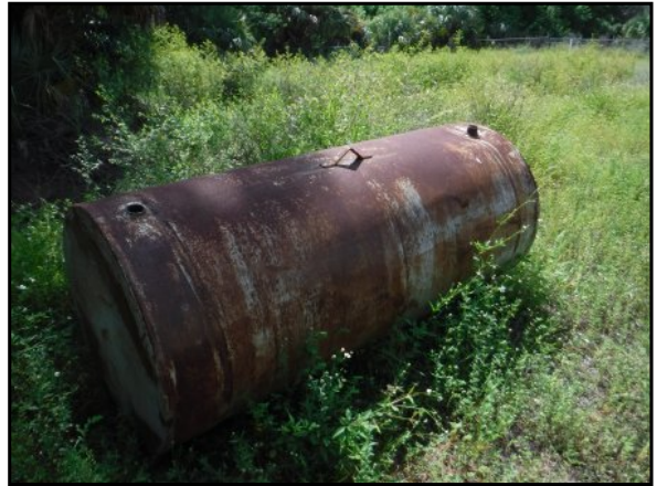
38 : Discarded abandoned diesel fuel AST
