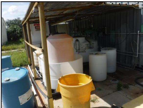
29 : Washing and waxing chemical storage canopy
