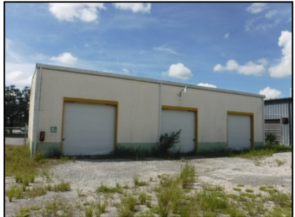
40 : Northern elevation of the storage building
