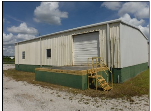
52 : Warehouse building, looking northwest
