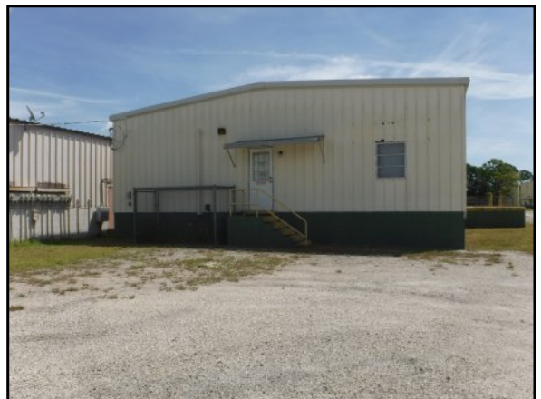
60 : western elevation of the warehouse building
