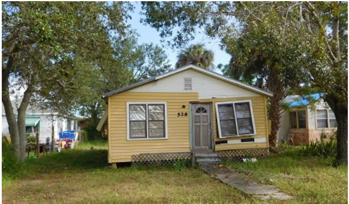
Structure to be demolished View from N 12th Street
