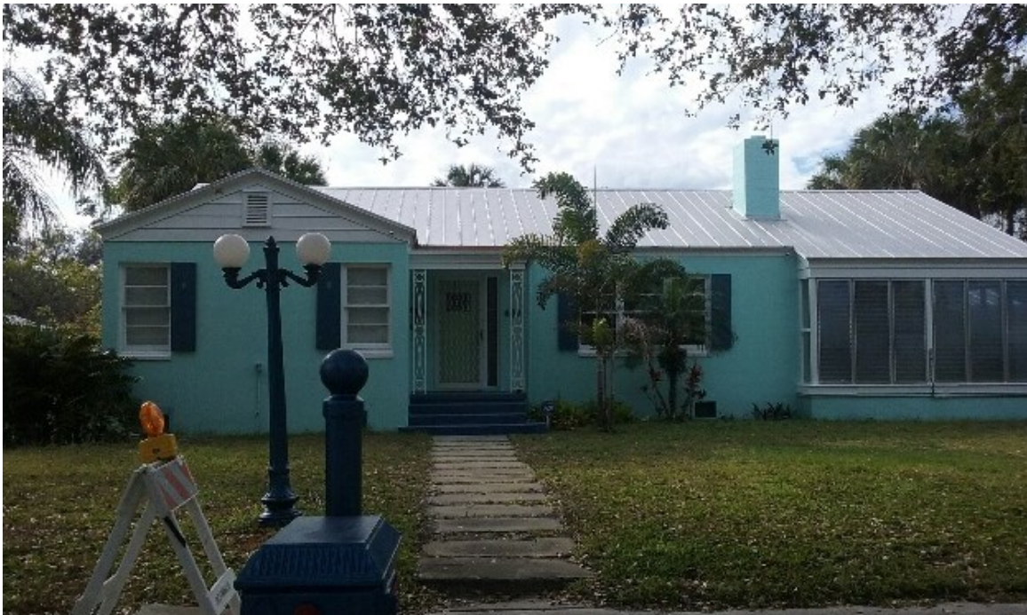
8th Street façade
