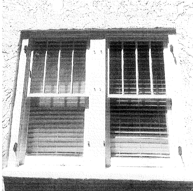
Windows and door proposed for replacement
