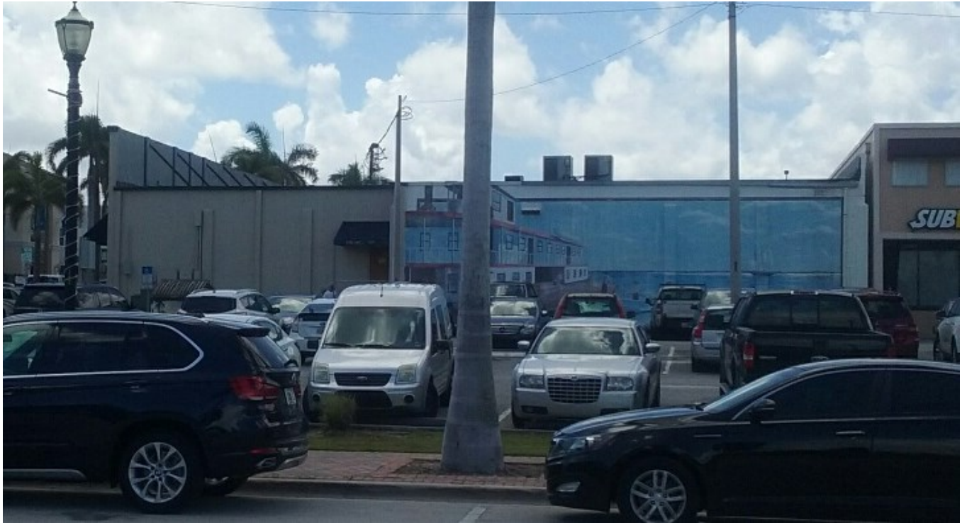
Existing Indian River Drive Façade
