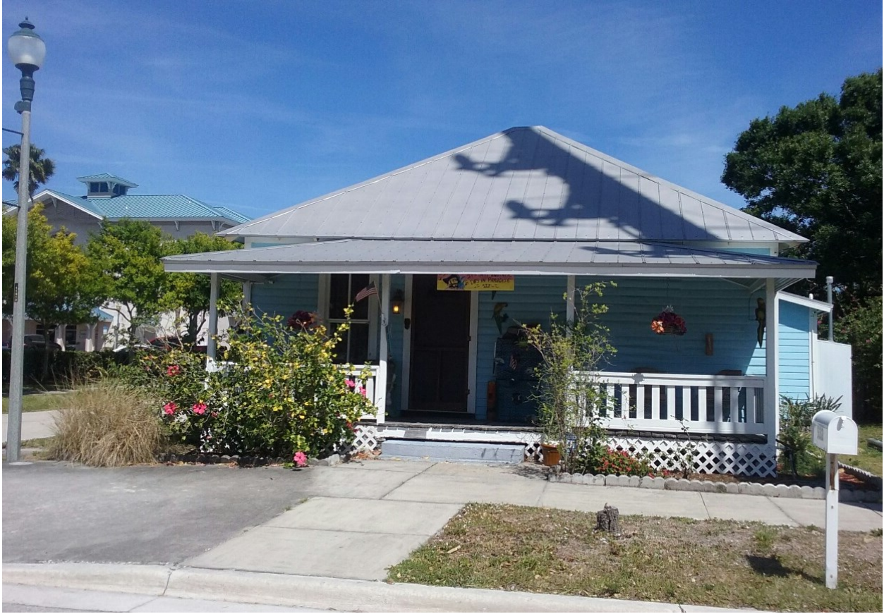
Front Façade of the Existing Residence
