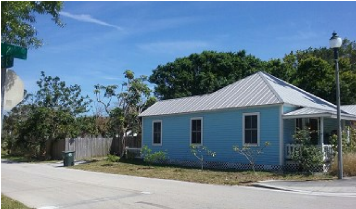
Side/Avenue E Façade of the Existing Residence
