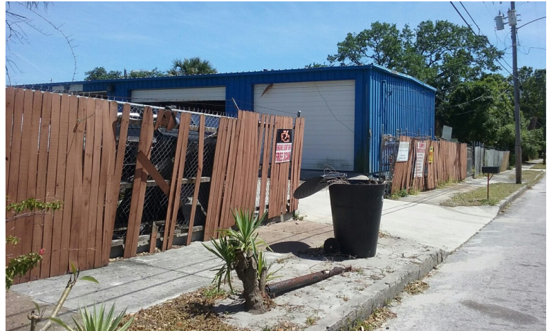
Existing fence east side of the N 6th street
