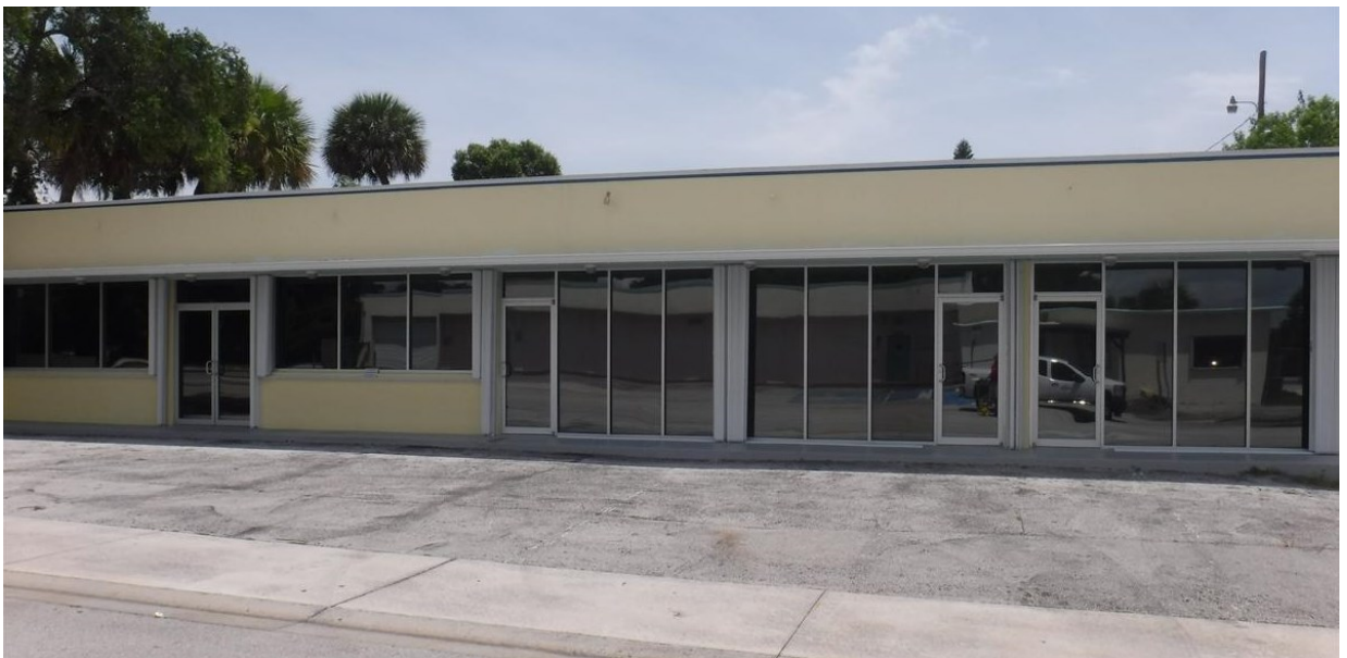
Front / 7th Street Facade
