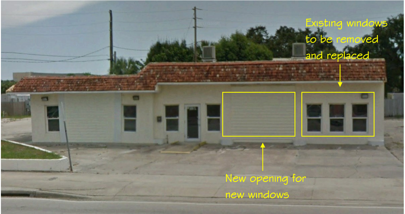
Existing US Highway 1 Façade
