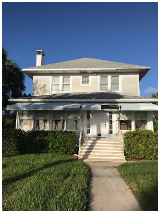
S Indian River Drive facade
