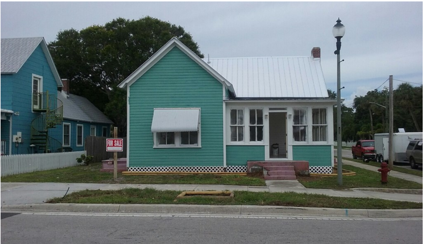
Existing Façade Fronting 7th Street
