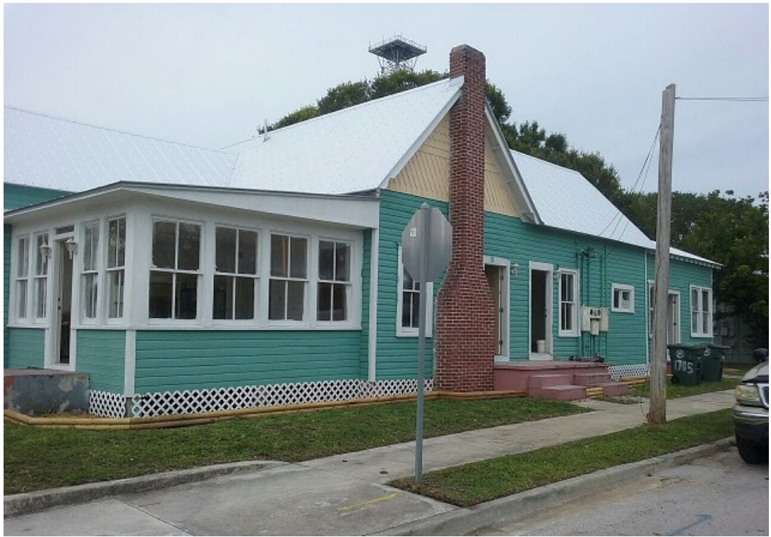
Existing Façade Fronting Boston Avenue
