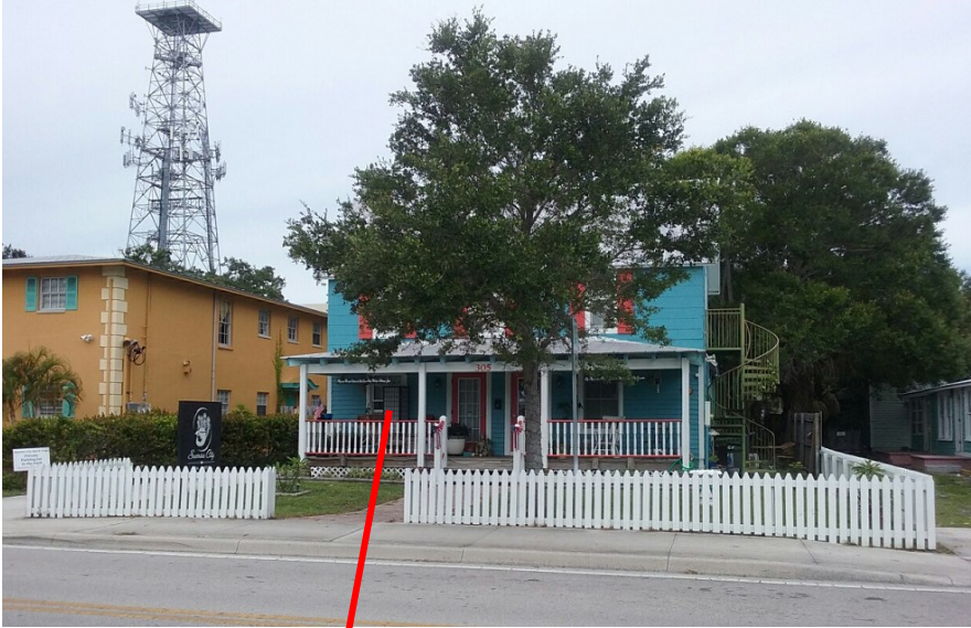
305 S 7th Street Front Façade Existing Fence
