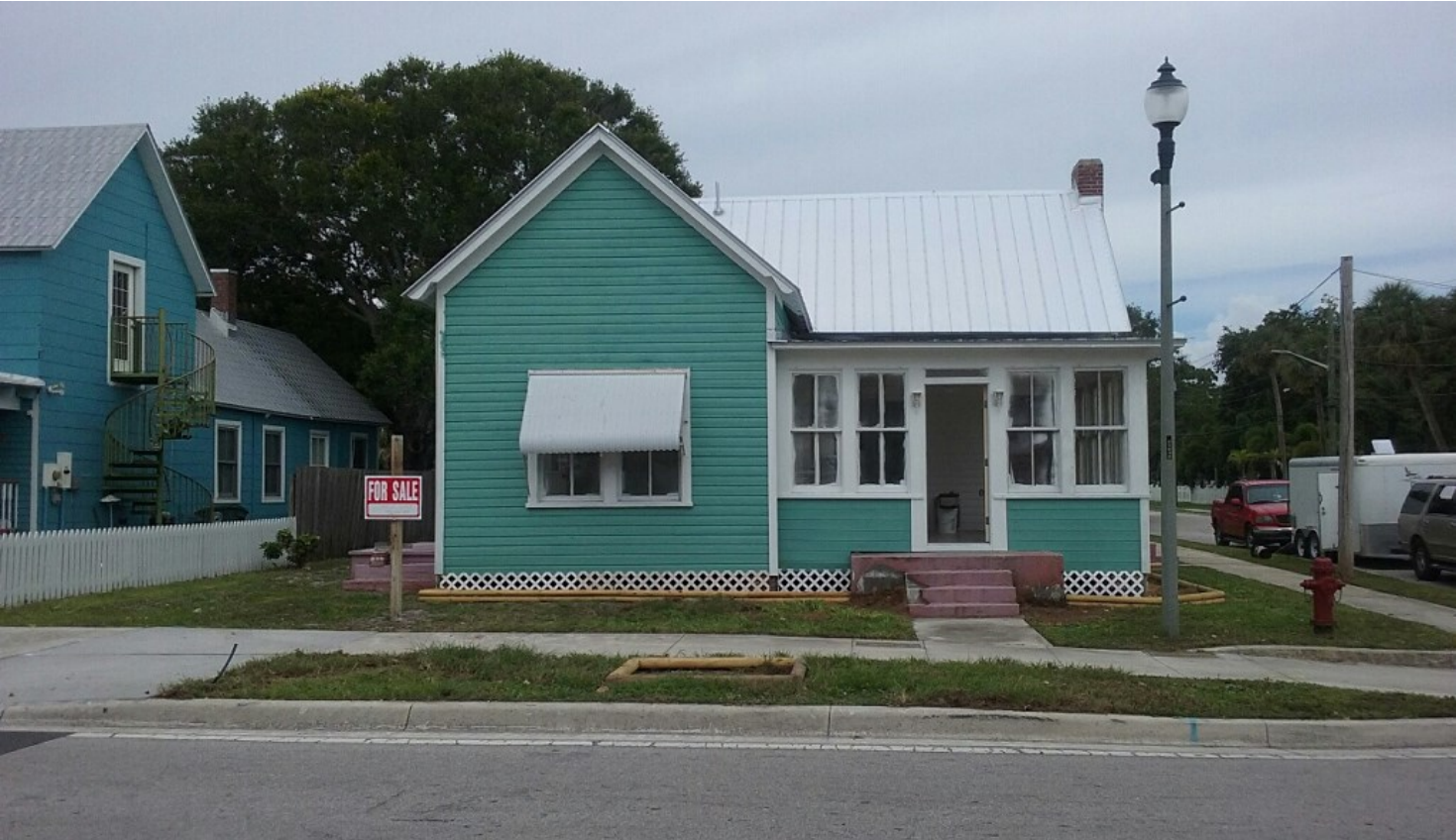
Existing Façade Fronting 7th Street
