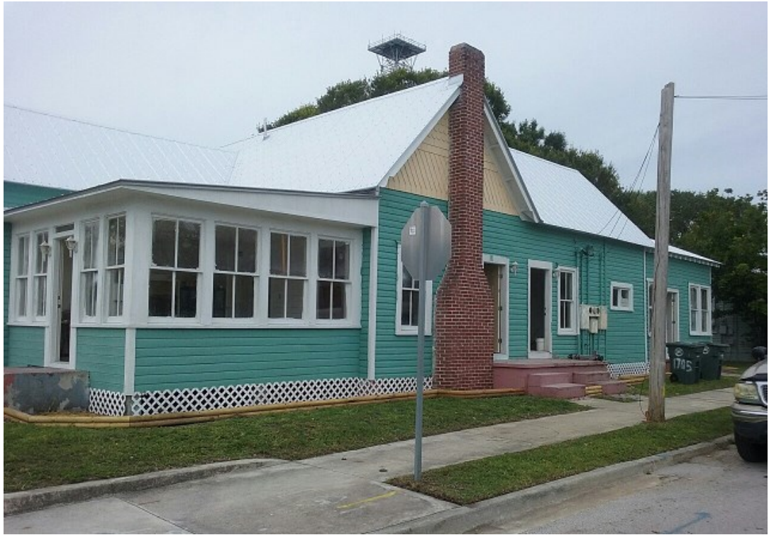
Existing Façade Fronting Boston Avenue
