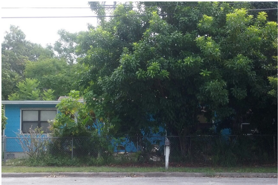
Side/S 8th Street Façade of the Existing Residence
