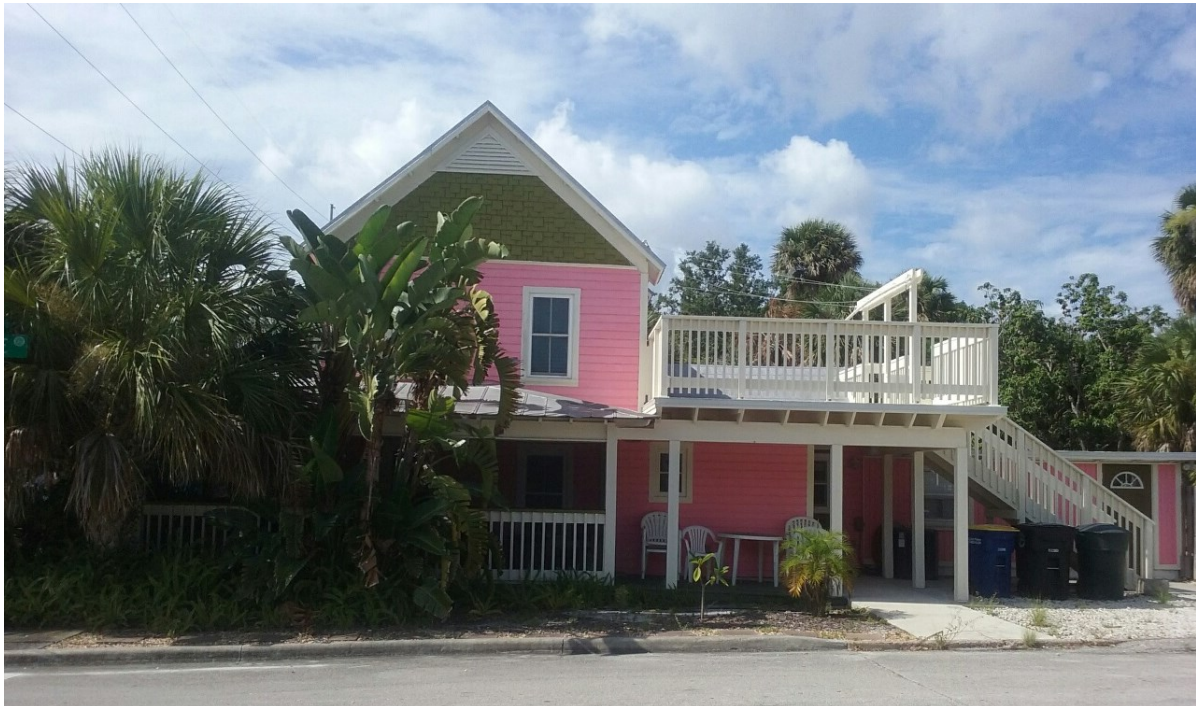
Side/Avenue E Façade of the Existing Building
