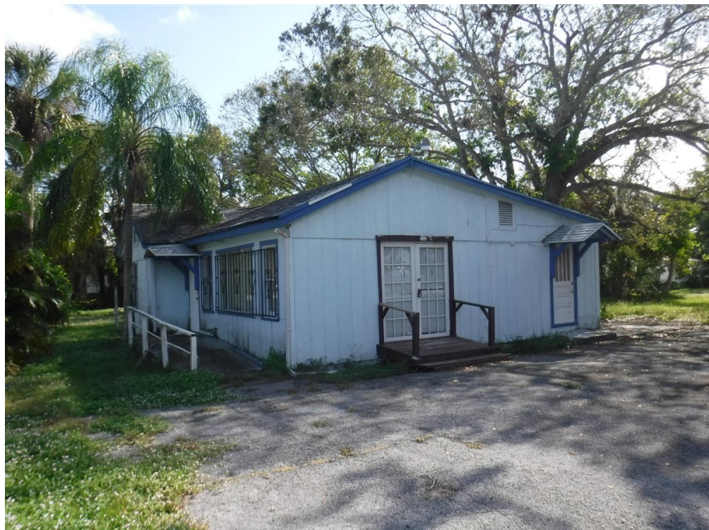
10th Street façade
