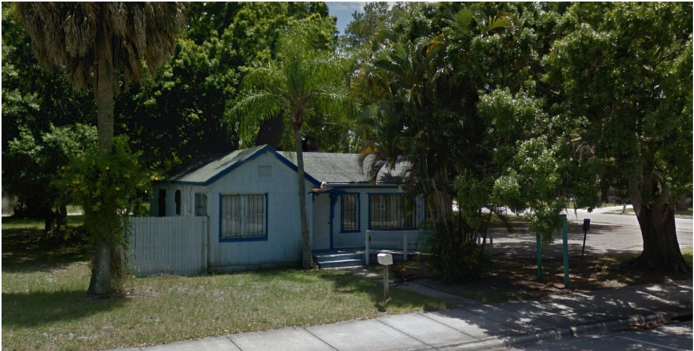
Delaware Avenue façade
