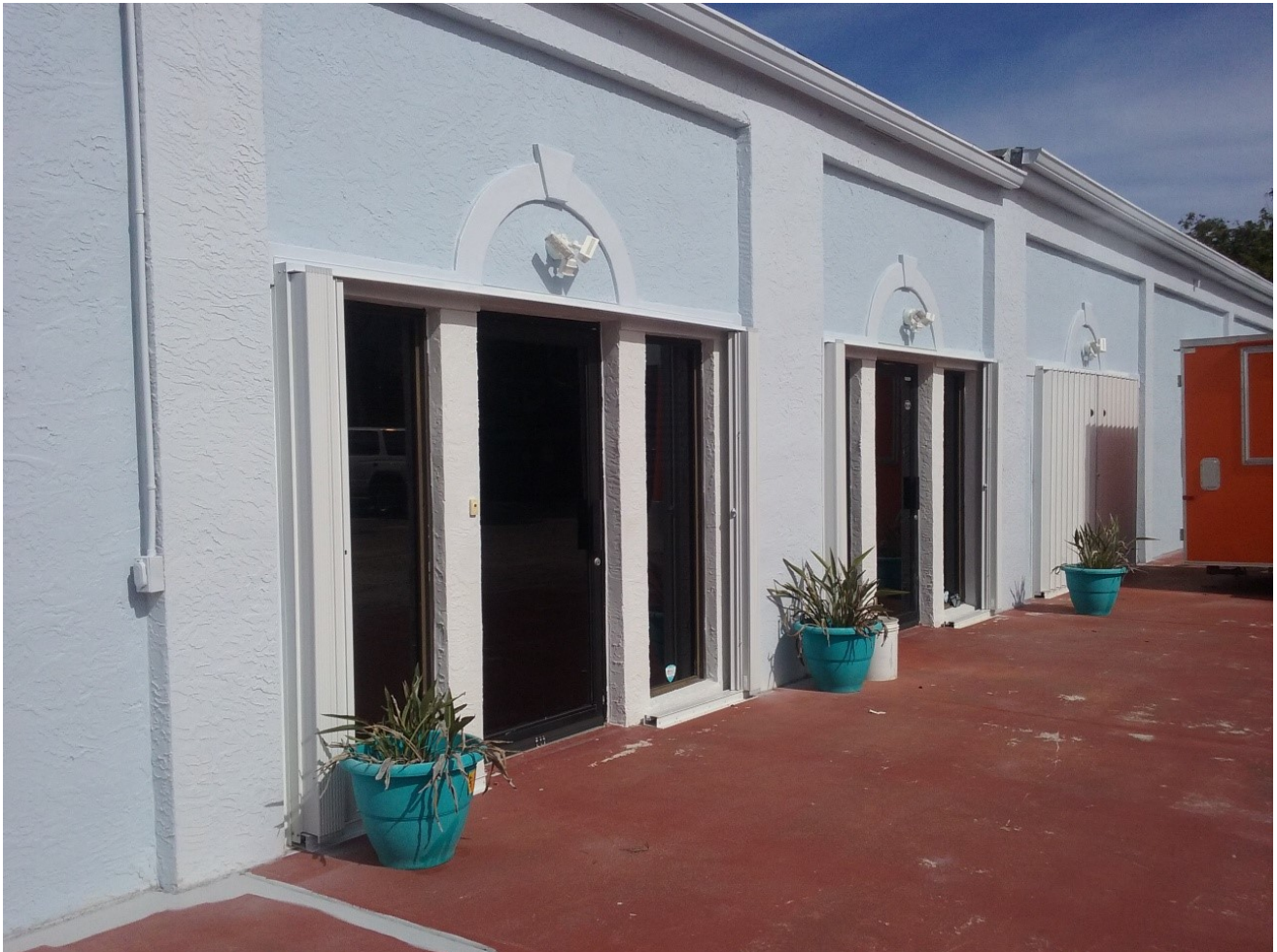
Example of accordion shutters mounted on the building at 218 N 2nd Street in Downtown area.
