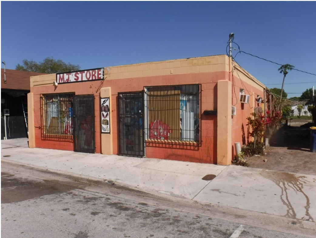
Avenue D facade
