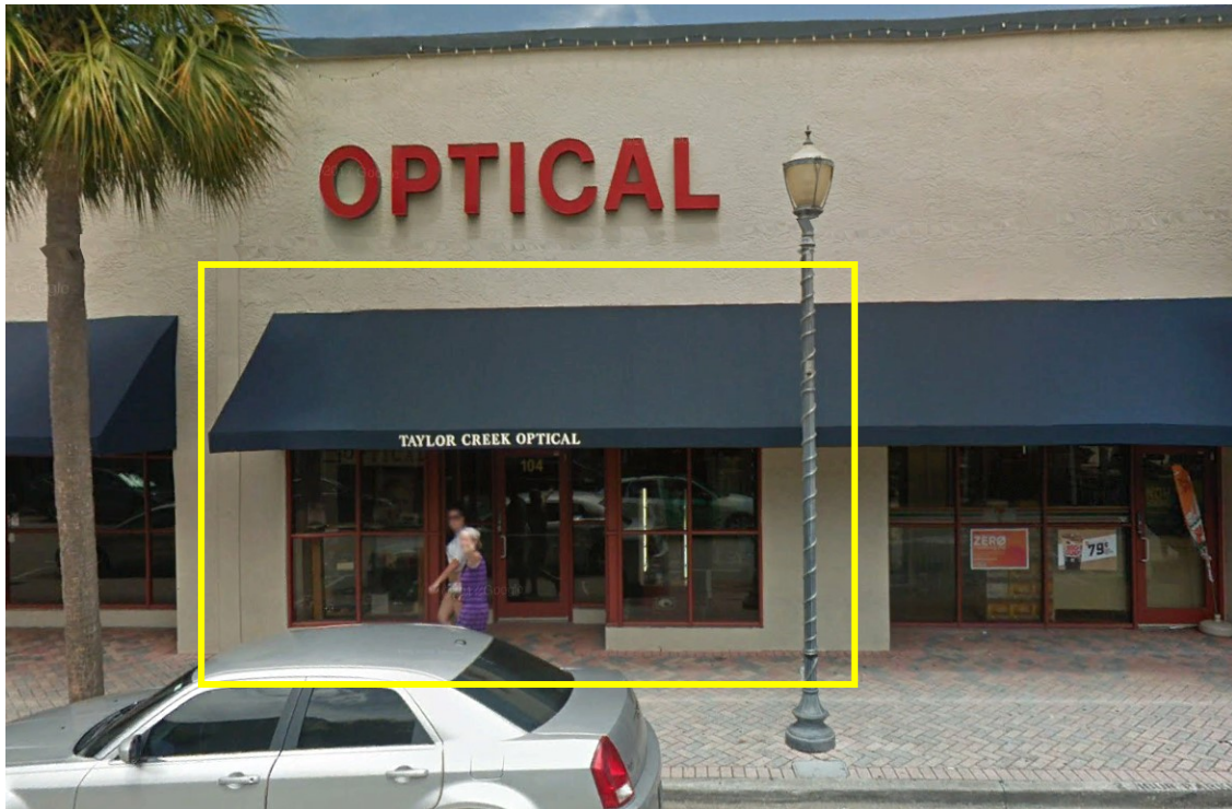
2nd Street Façade/Subject Window
