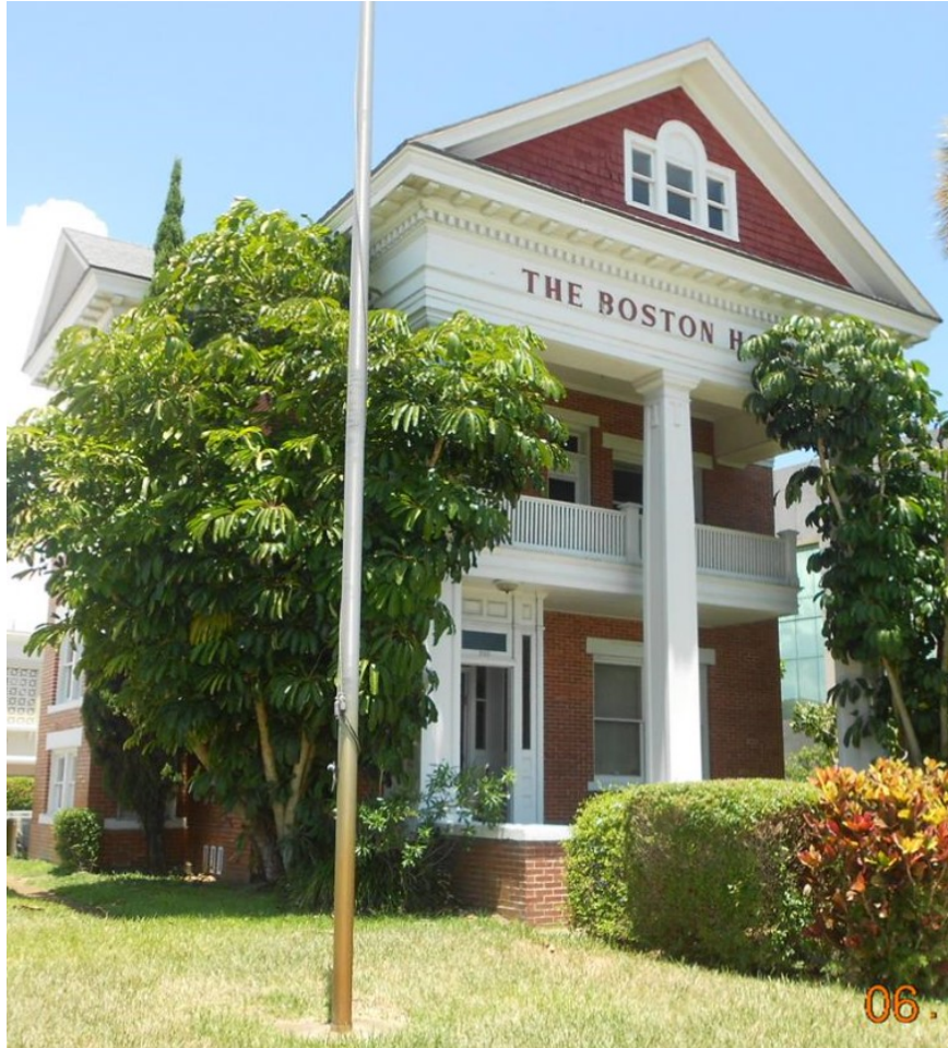
Front/Indian River Drive Façade
