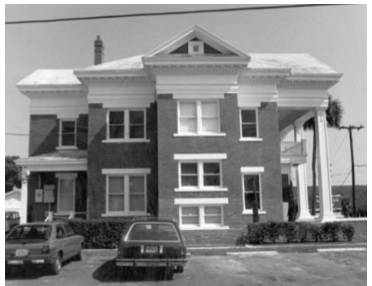
South Side Façade
