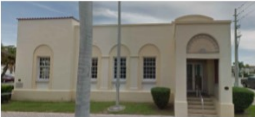
STREET VIEW (SOUTH FACADE)
