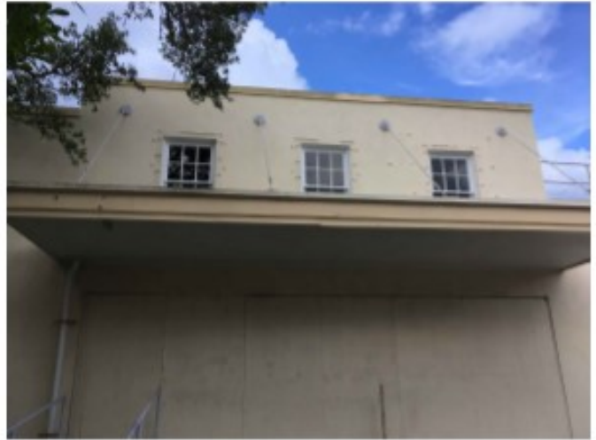
CLOSE UP OF NORTH FACADE OVERHANG
