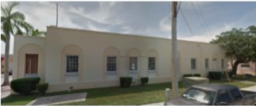
STREET VIEW (EAST FACADE)
