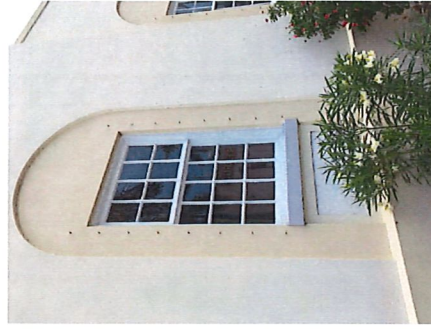
CLOSE-UP OF WINDOW
