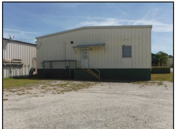
60 : western elevation of the warehouse building
