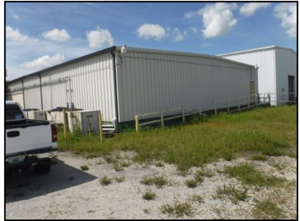
50 : Overview of citrus processing building, looking southwest
