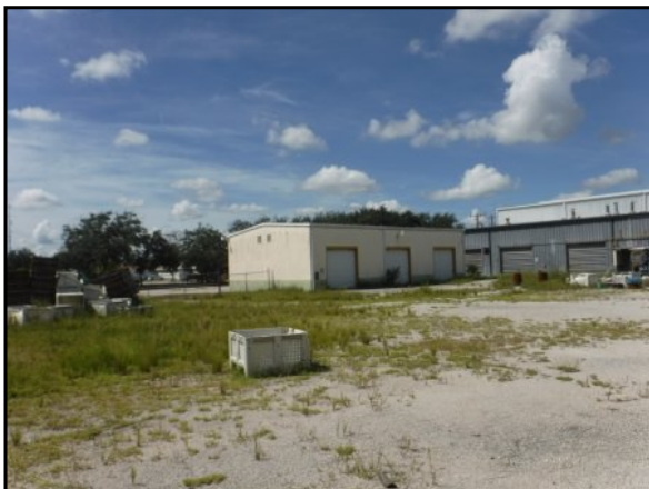
35 : Storage building, looking southwest
