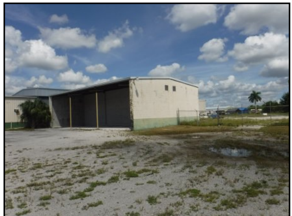
66 : Eastern elevation of the storage building
