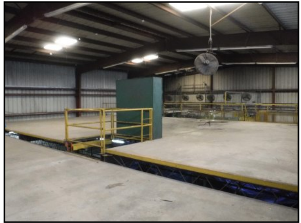
16 : Mezzanine area (second floor) in citrus processing building
