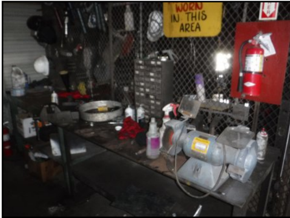
7 : Maintenance area of the citrus processing building
