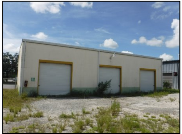
40 : Northern elevation of the storage building
