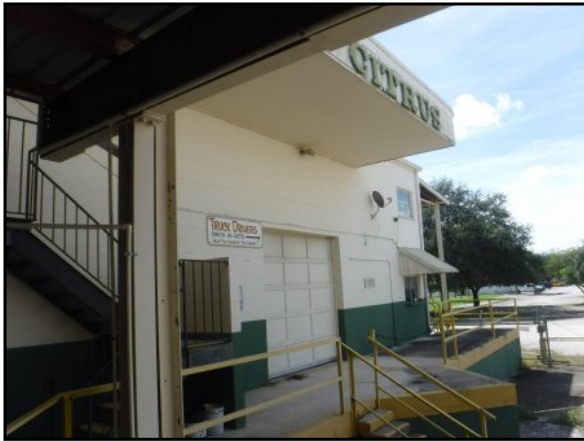
21 : Loading dock area for the citrus processing building
