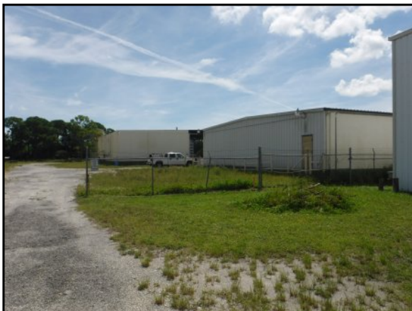
53 : Property overview, looking east
