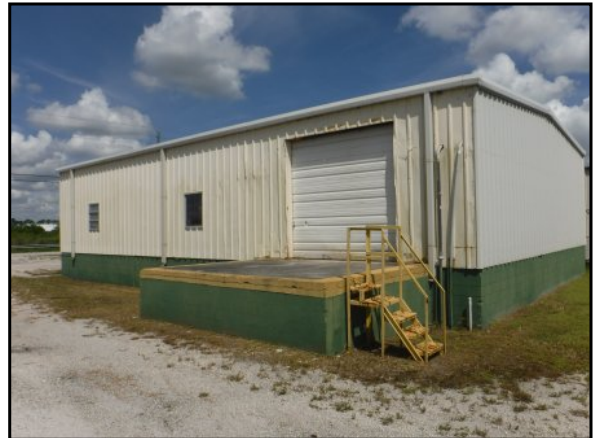
52 : Warehouse building, looking northwest
