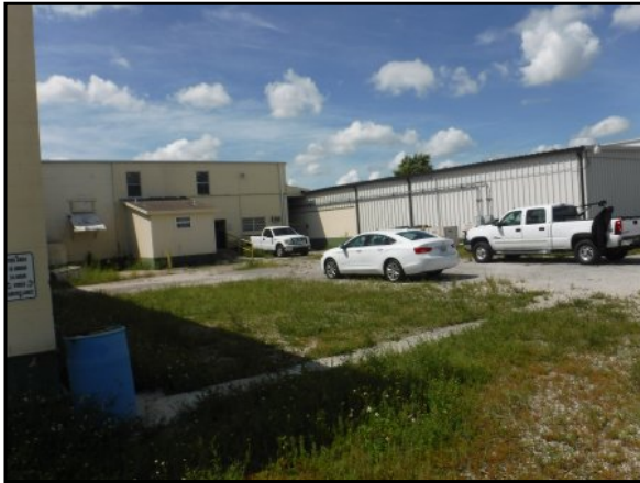
49 : Overview of citrus processing building, looking south
