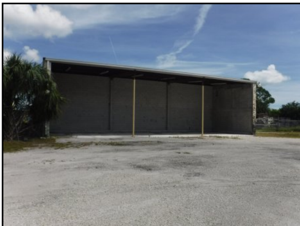
65 : Southern elevation of the storage building
