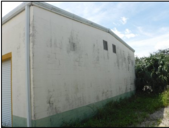
45 : Western elevation of the storage building
