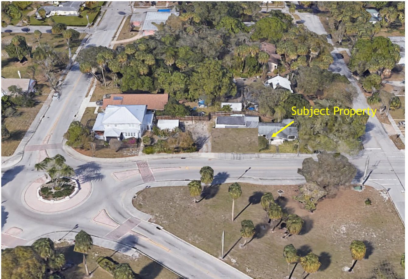
Aerial view of the property
