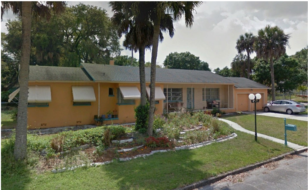
Easter Avenue/North Façade
