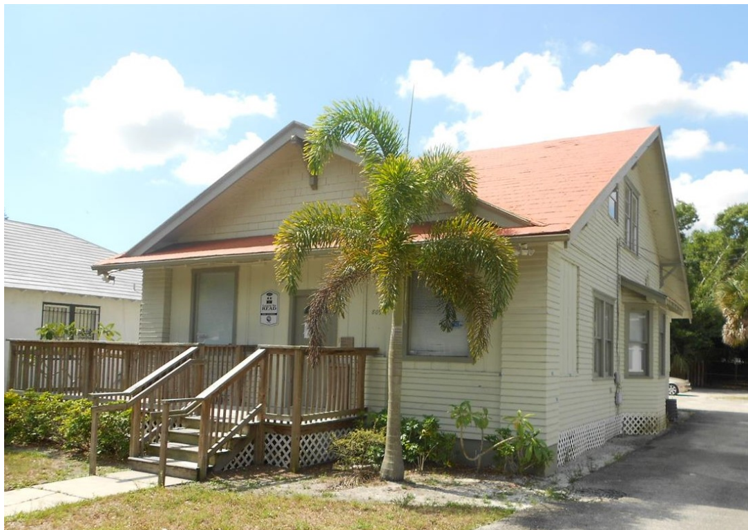
Delaware Avenue Façade
