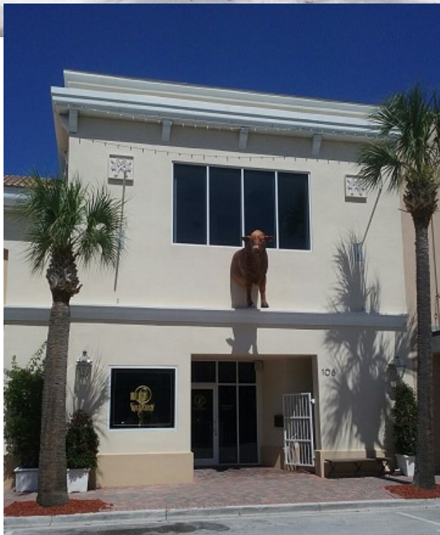
Existing Front Façade
