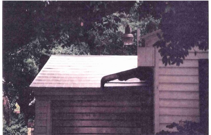
Existing roof material metal shingles
