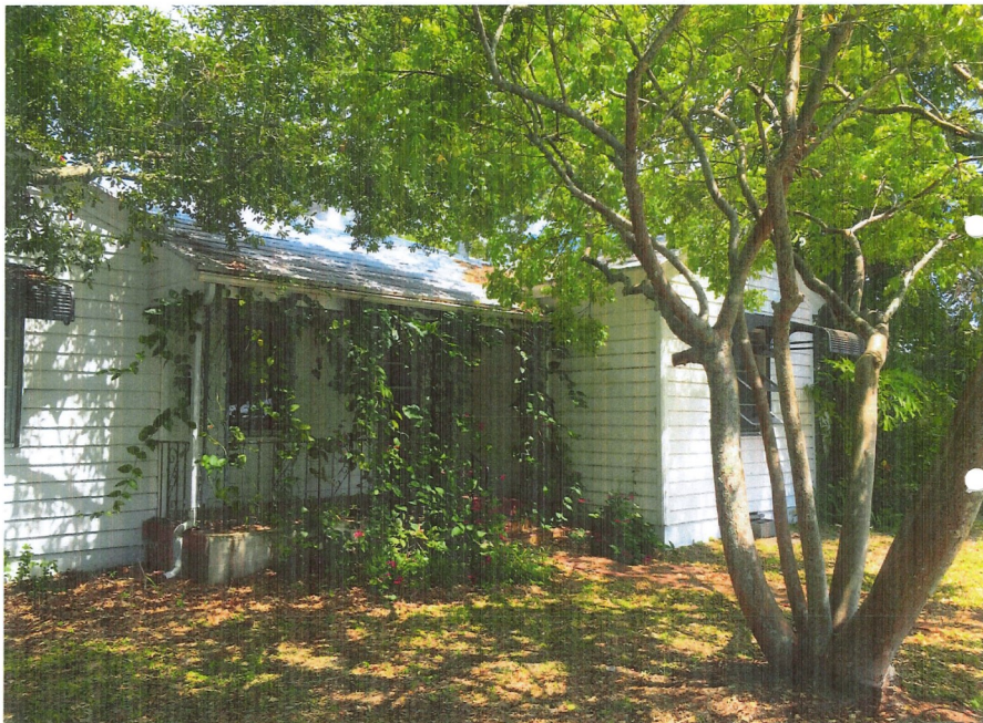
Rear façade of the residence
