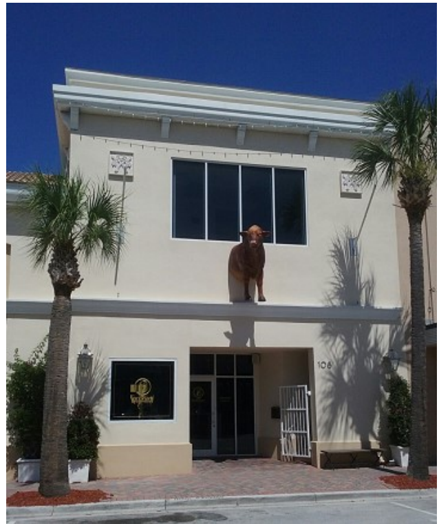
Existing Front Façade
