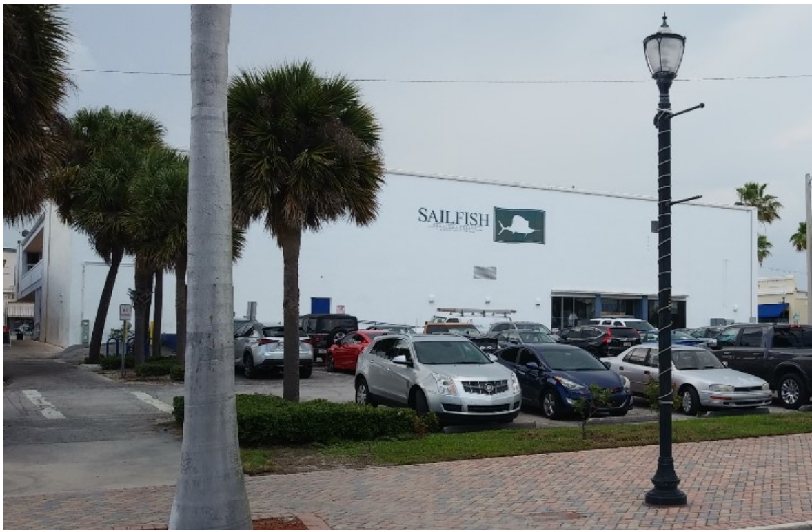
Existing Façade of the Building
