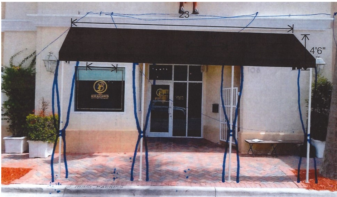
Placement of the poles inside proposed drapes.
