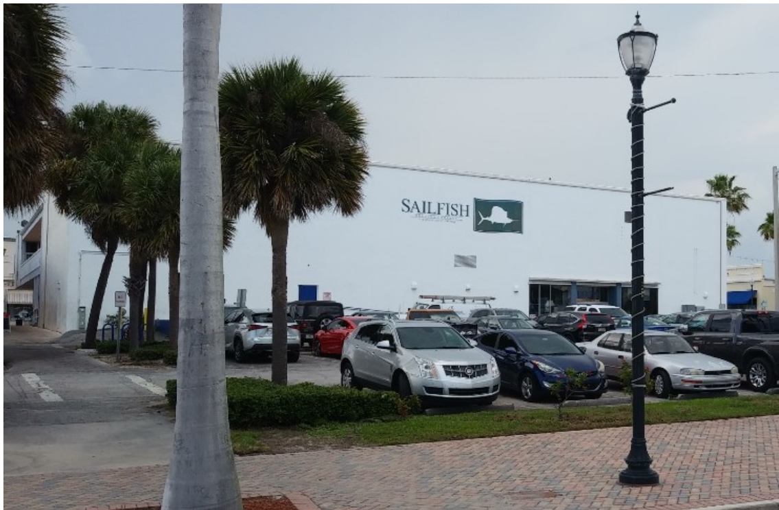
Existing Façade of the Building
