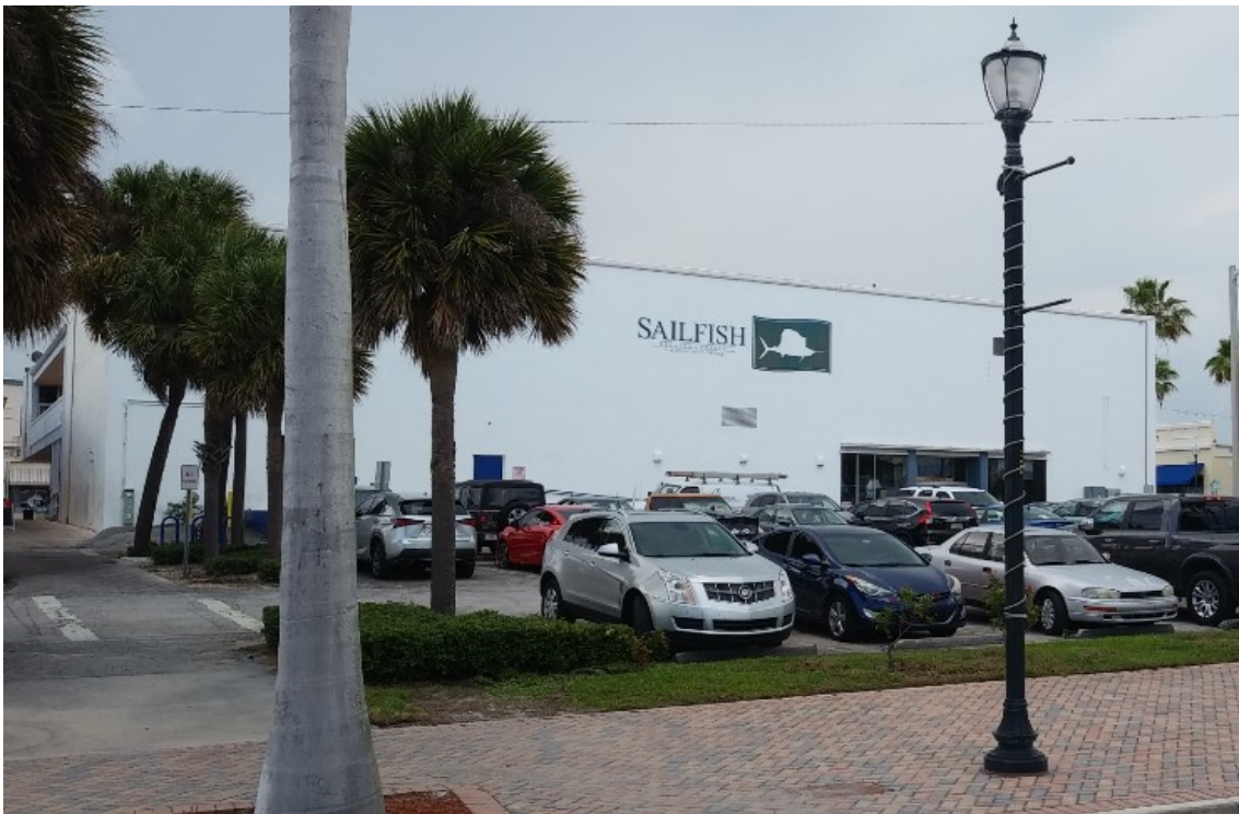
Existing Façade of the Building
