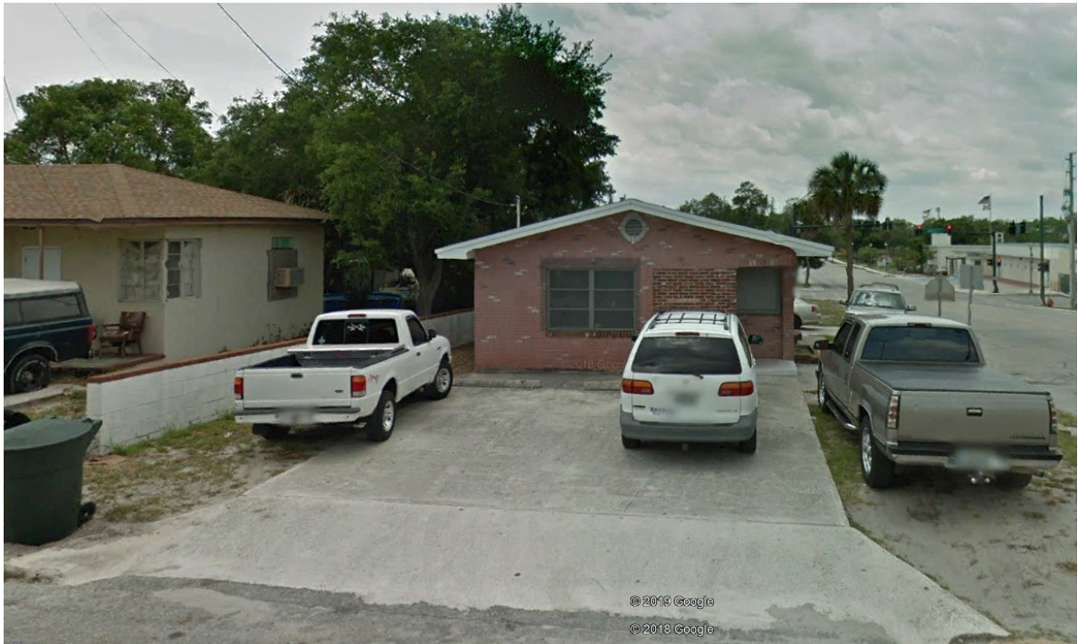
View from Cedar Place/side of the property
