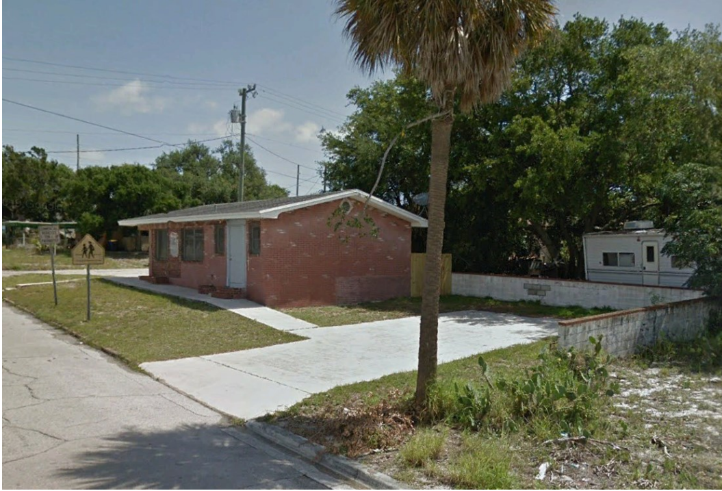
View from 7th Street/front of the property
