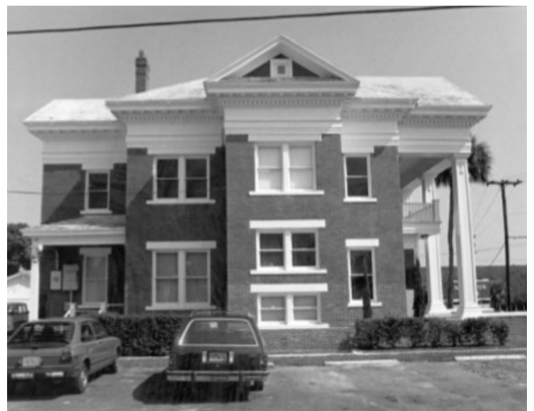
South Side Façade
