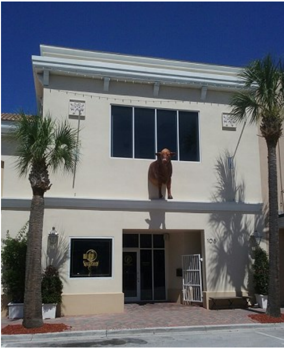
Front view with the existing sign
