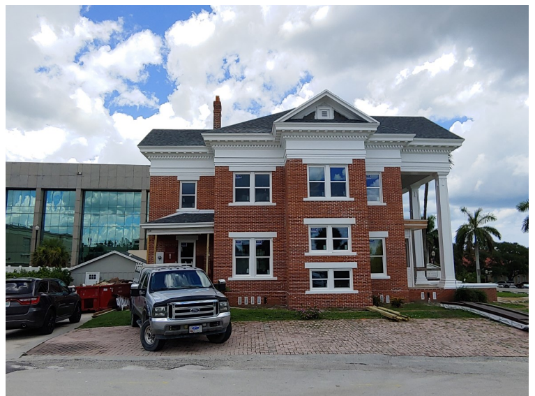
South Side Façade
