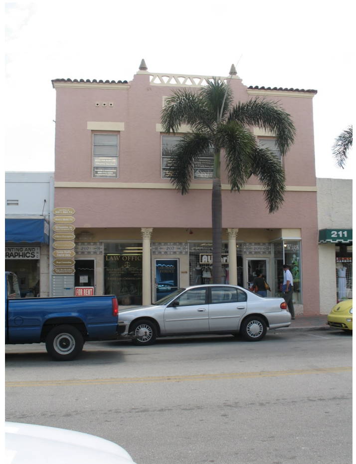
Front/Orange Avenue Façade 2007
