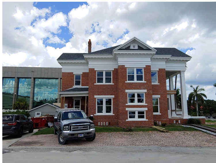
South Side Façade
