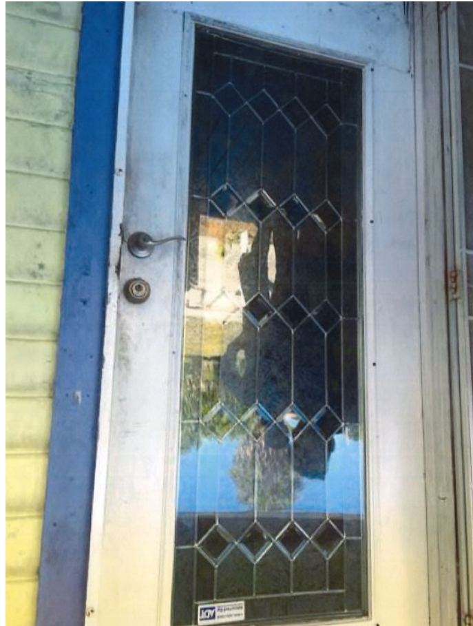
Doors proposed for replacement.
