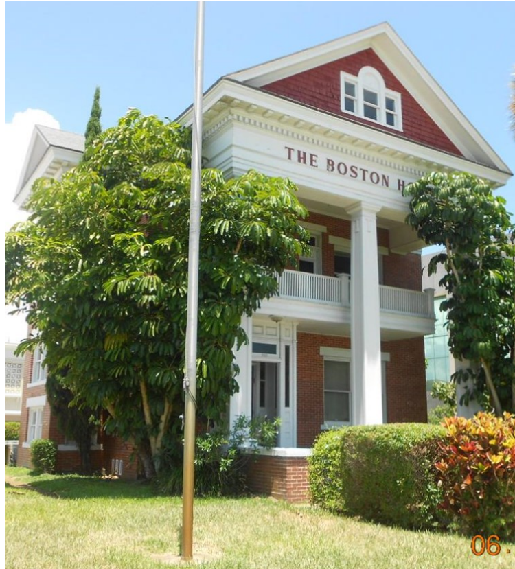
Front/Indian River Drive Façade
