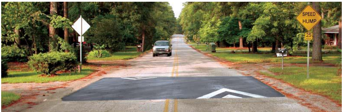
Exhibit 3.1 - Typical Speed Hump Application:
