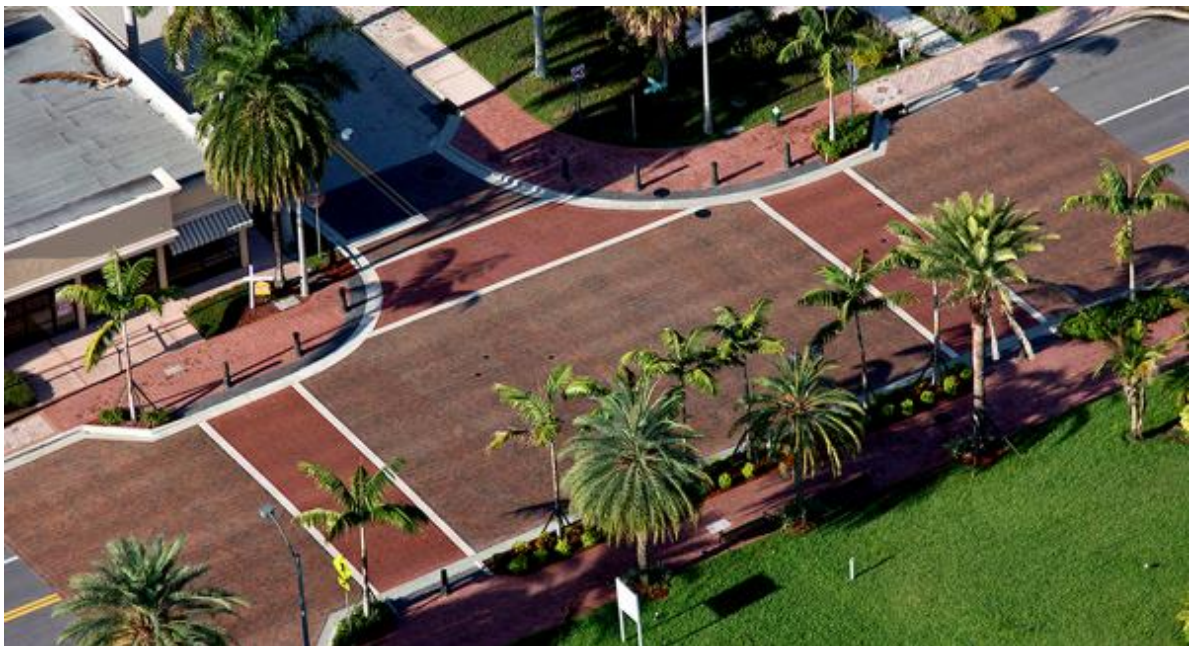
Exhibit 3.3 - Typical Speed Hump Application:
